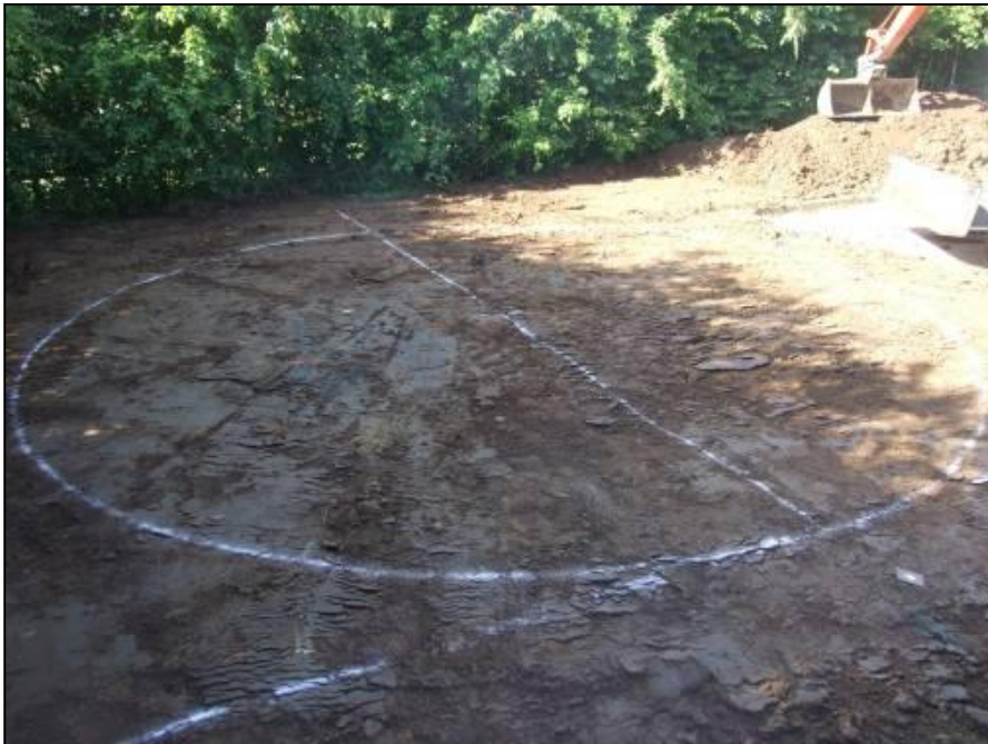
PLATE 2: Pre excavation shot of balance tank area
