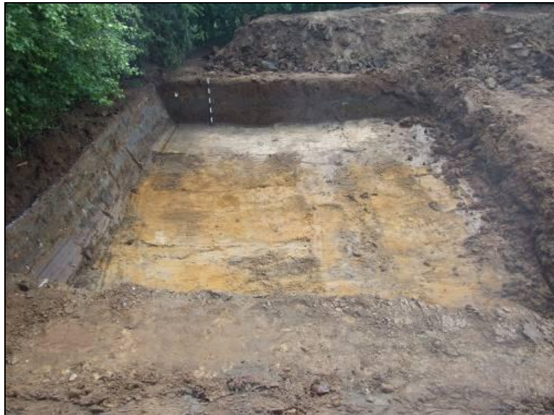
Overview of excavated area looking north
