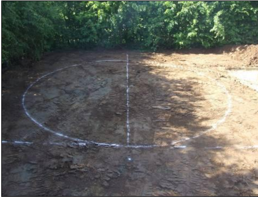
PLATE 1: Pre excavation shot of balance tank area looking north
