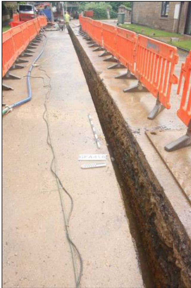
Plate 15: Representative section of vacuum sewer trench on Main Street, looking east
