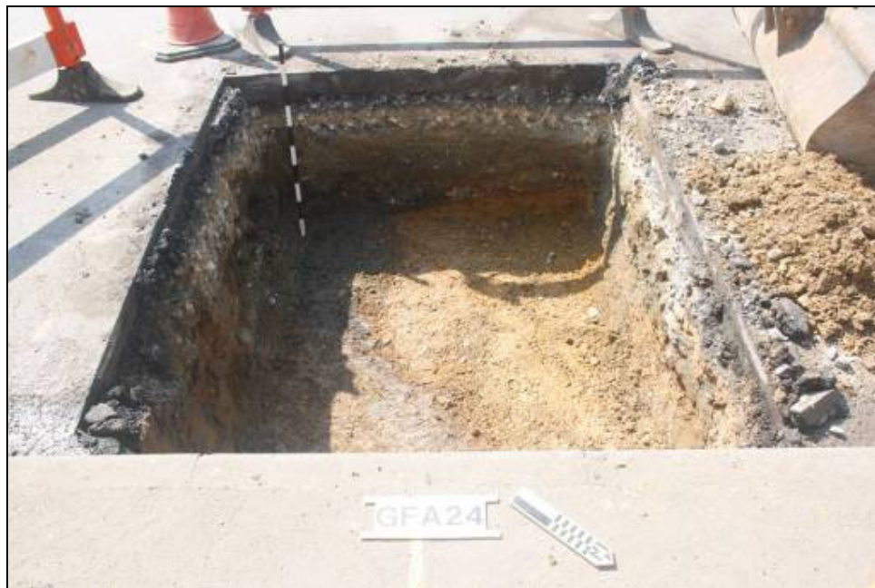
Plate 5: Pot #24 looking north-west, showing north-south aligned ditch [1078]
