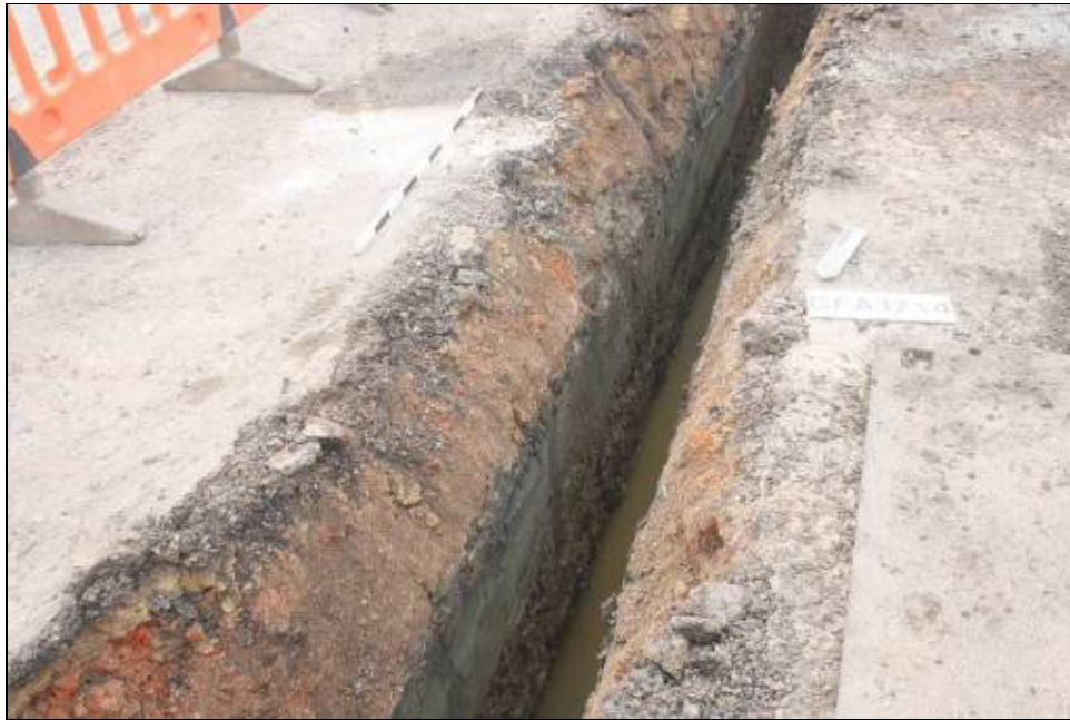
Plate 8: Representative section of vacuum sewer trench in Greatford Gardens, looking south-east
