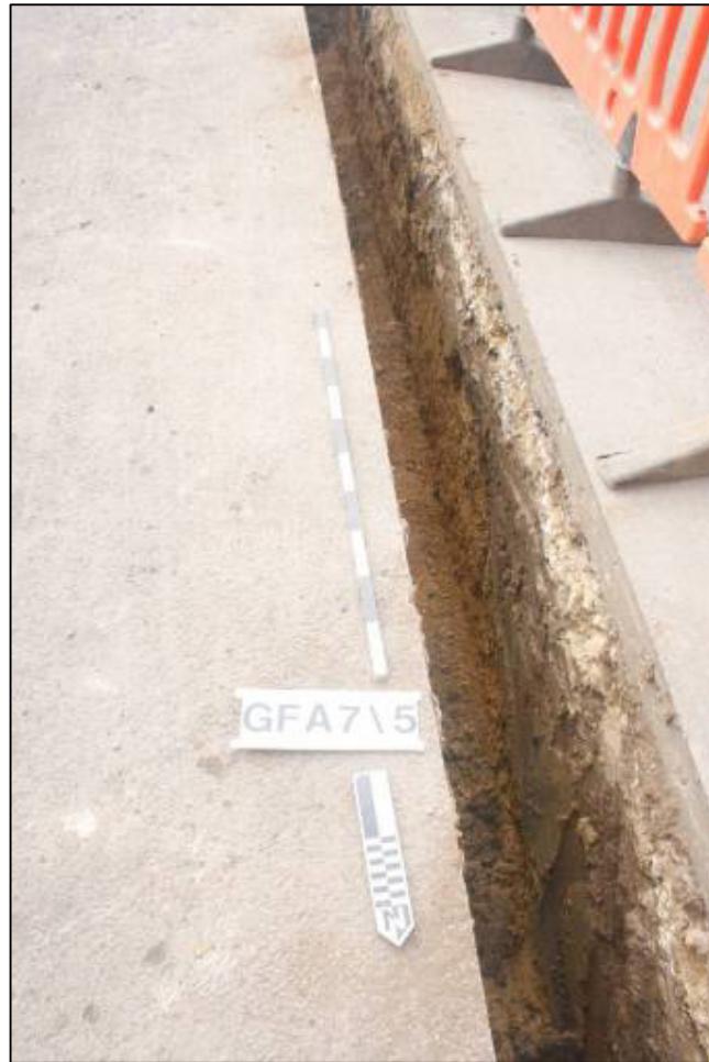
Plate 9: Representative section of vacuum sewer, south of the West-Glen River
