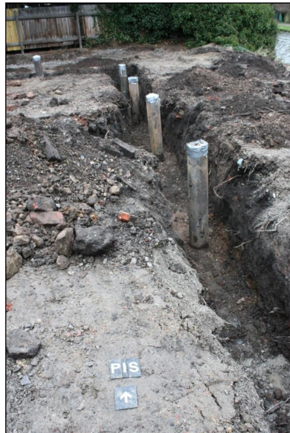
Plate 24: Shot of finished trenches
