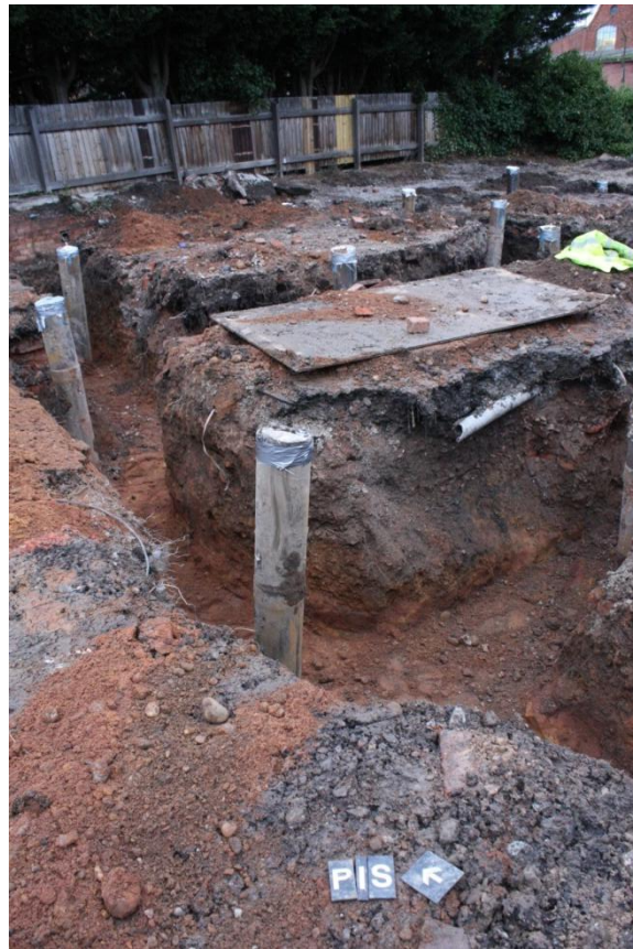
Plate 23: Shot of finished trenches
