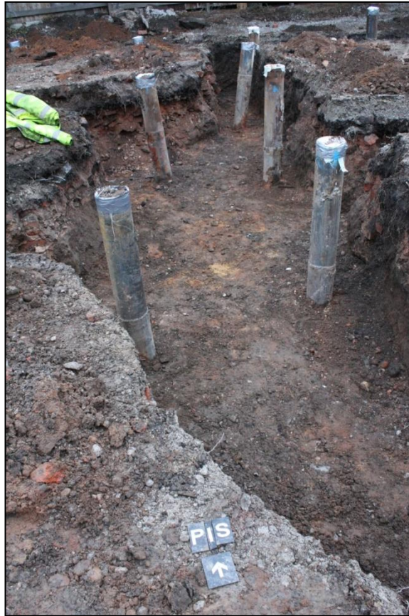
Plate 25: Shot of finished trenches
