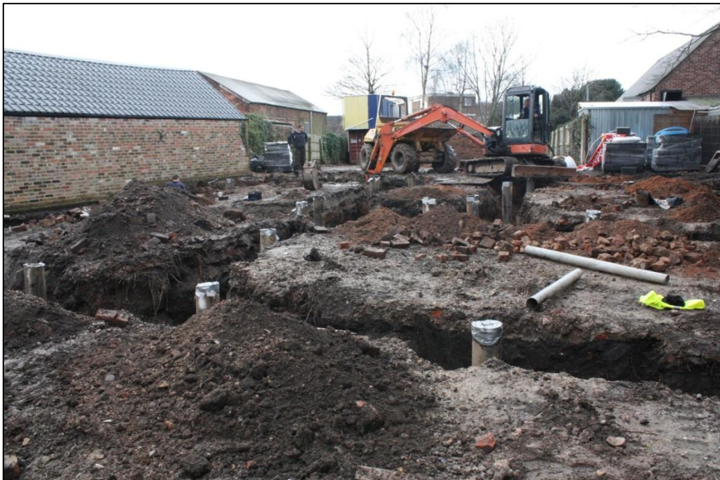
Plate 20: General shot, looking south west
