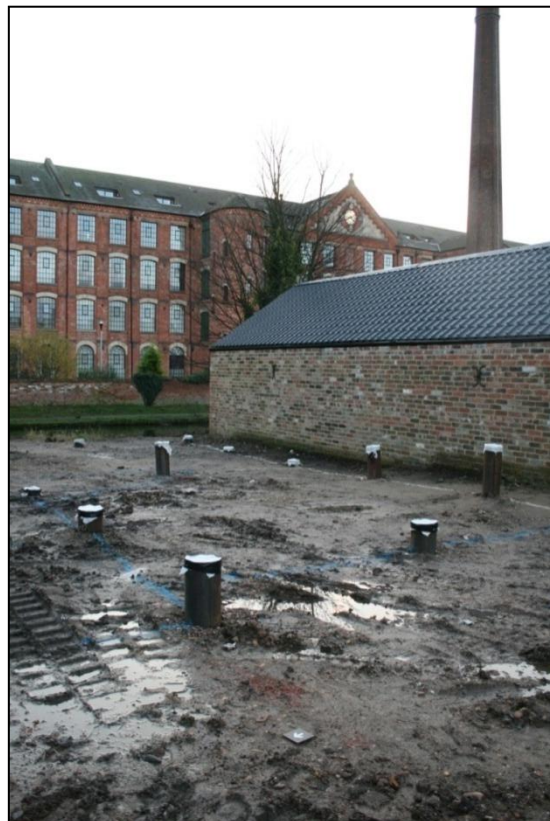
Plate 4: Eastern trench adjoining the canal
