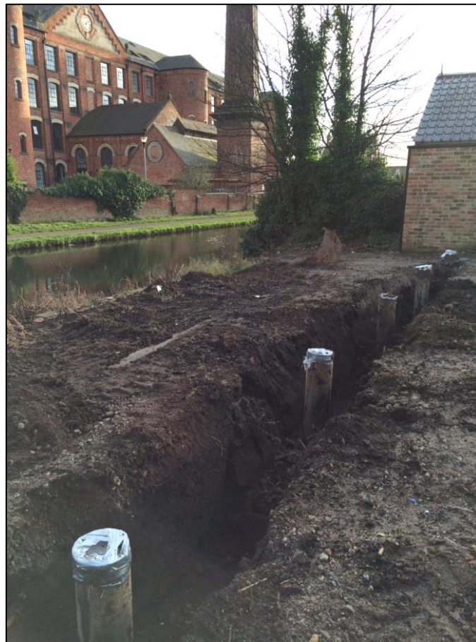
Plate 2: General shot of site pre excavation with adjoining grade listed building
