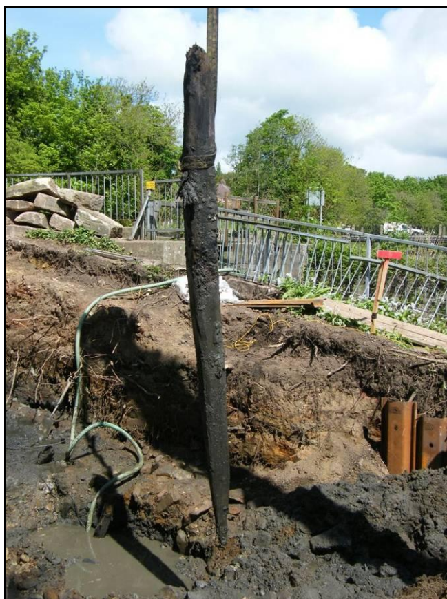
Plate 12. Photograph of timber after removal by machine excavator
