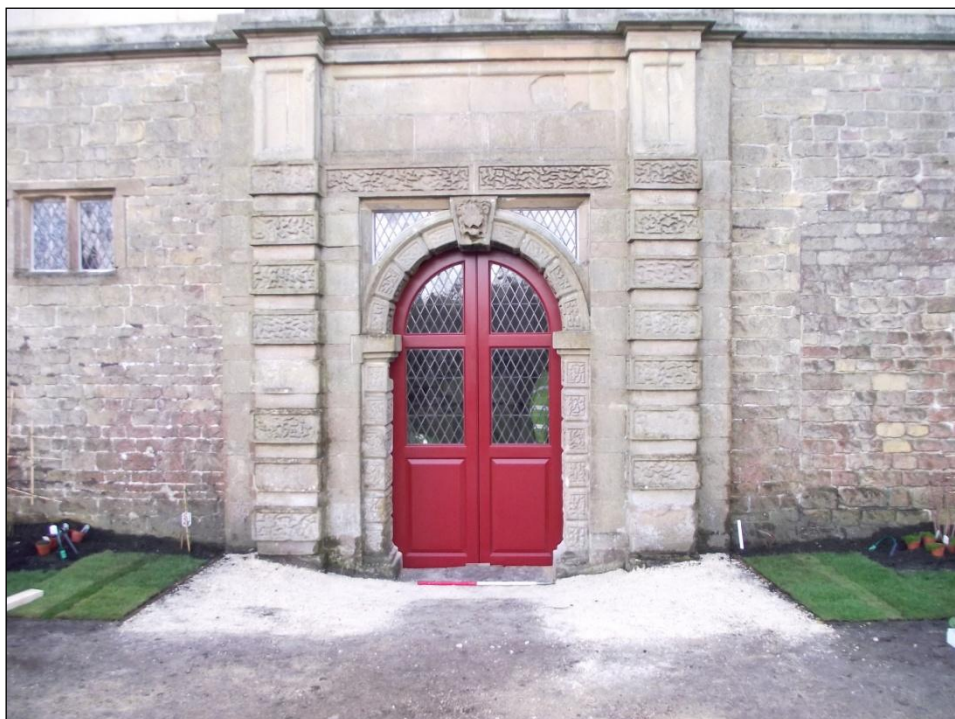
Plate 1. South looking photograph of West Garden Room
