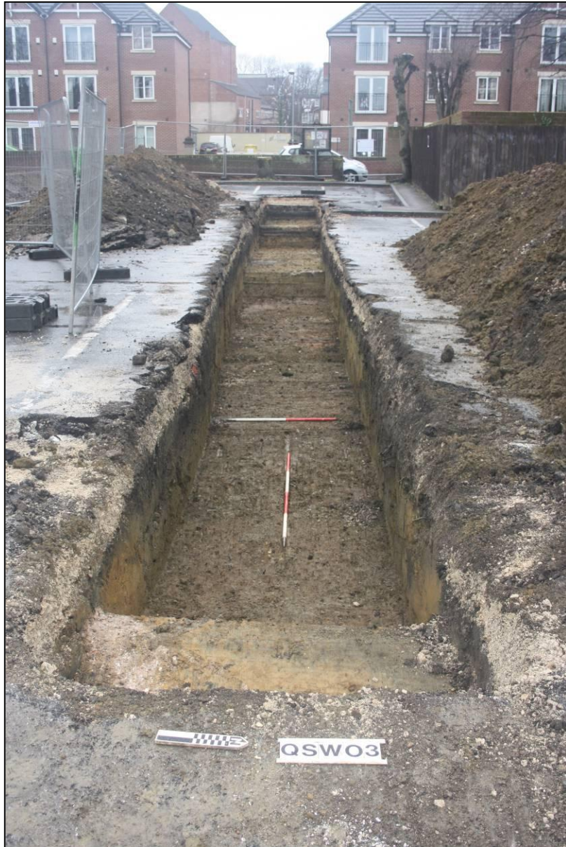
Plate 4: Trench 3 looking west, palaeochannel [0029] in foreground
