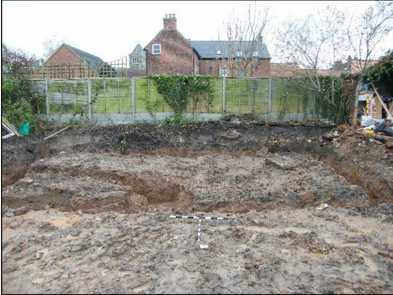
Plate 1: General view of the site with the former farmhouse, 48 Dennis Street, in the background, viewed looking north-west.
