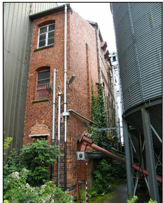
Plate 4: West corner of the maltings, viewed looking south-east.
