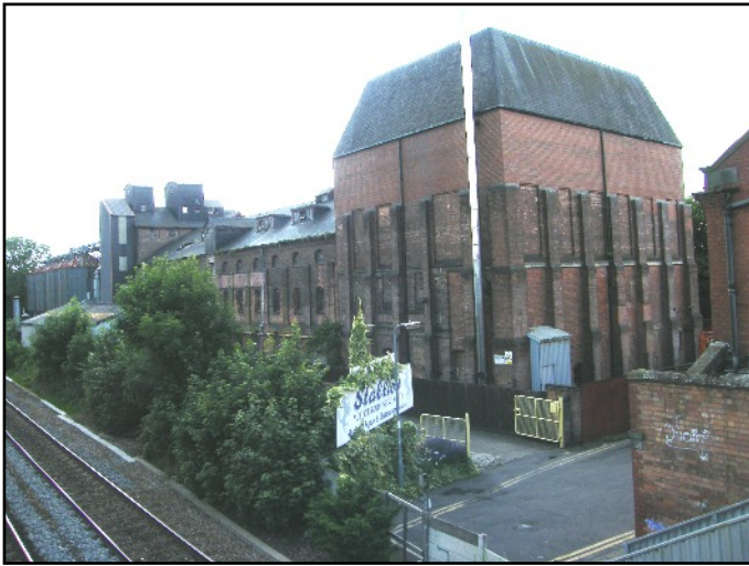
Plate 1: General view of Beeston Maltings, viewed looking west.
