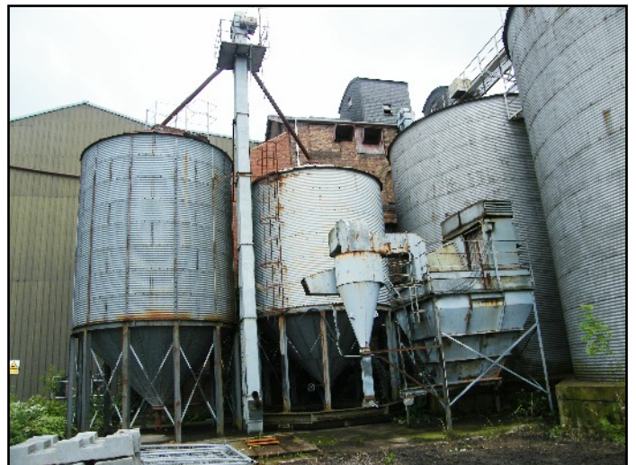
Plate 6: Modern silos located to the south-west of the maltings, viewed looking east.
