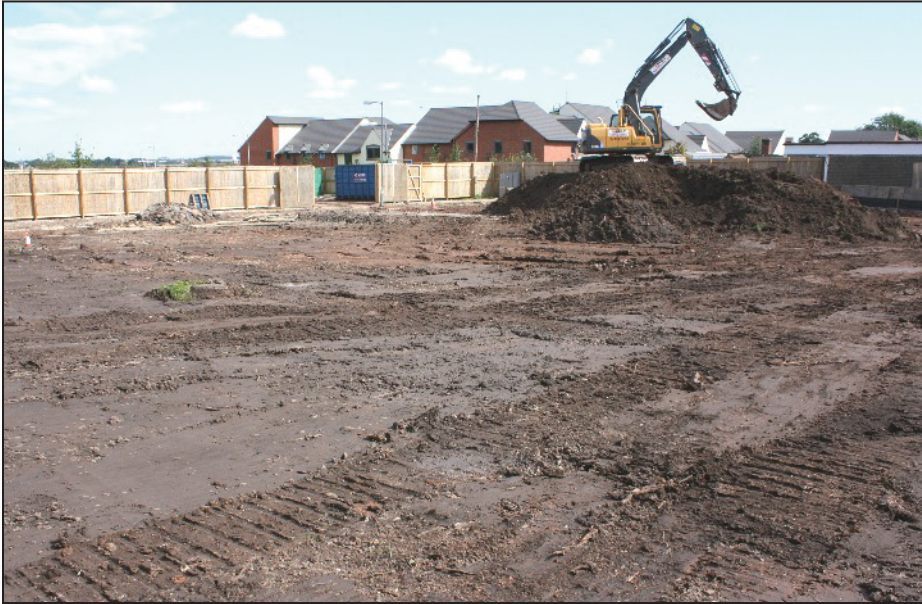
Plate 3: A later stage in the machine clearance of the library site.
