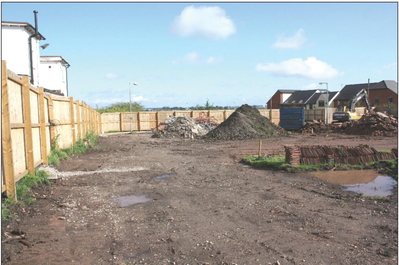
Plate 2: View looking north showing initial topsoil clearance.
