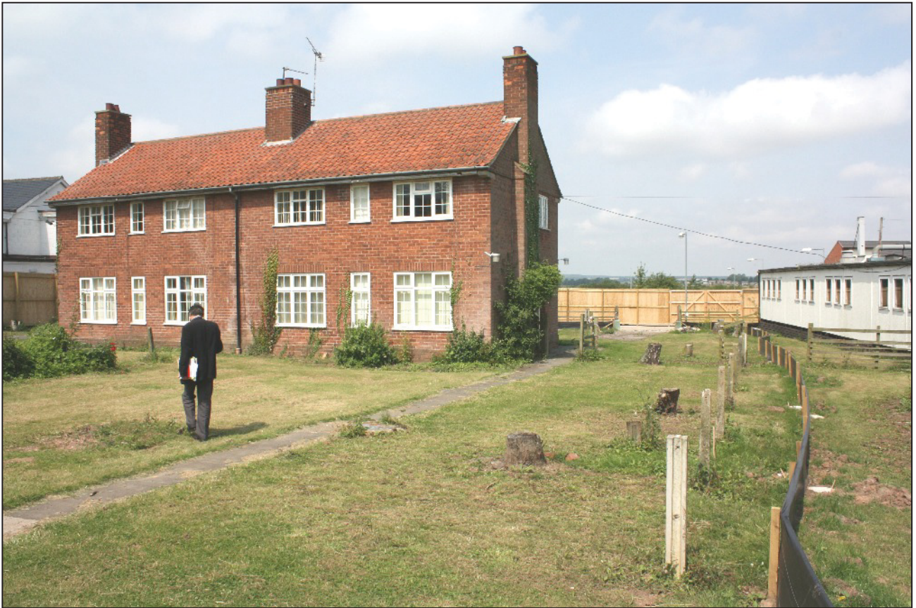
Plate 1: View of the site prior to the demolition showing the semi-detached houses and one of the two teaching blocks.
