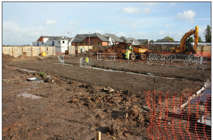
Plate 6: Infilled foundation trenches crossing the site.
