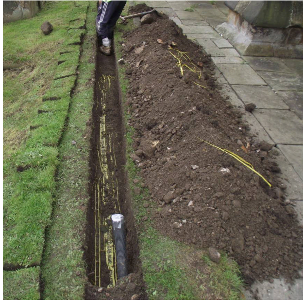
Plate 8: Area 05 during excavation. Looking south.
