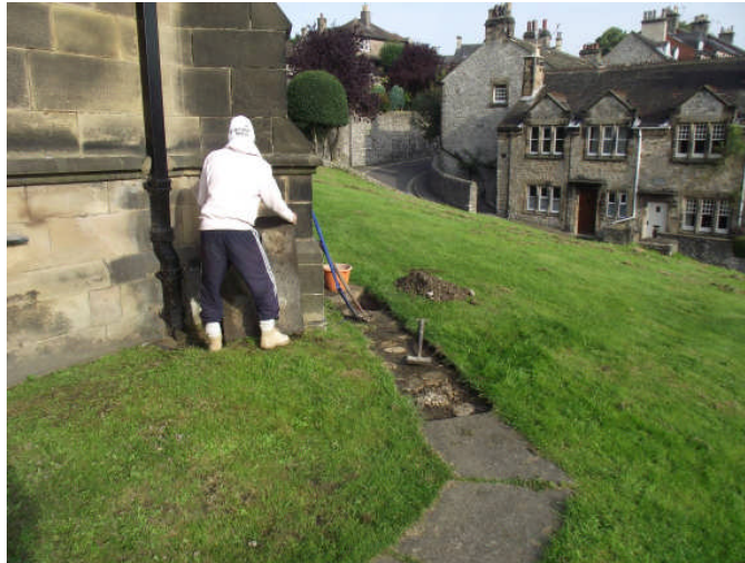
Plate 1: Paving slabs being removed prior to trenching in area 01. Looking north-west.
