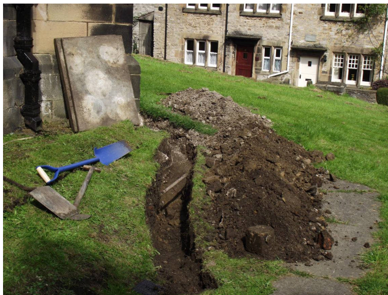
Plate 3: View of area 01 fully excavated. Looking north-west.
