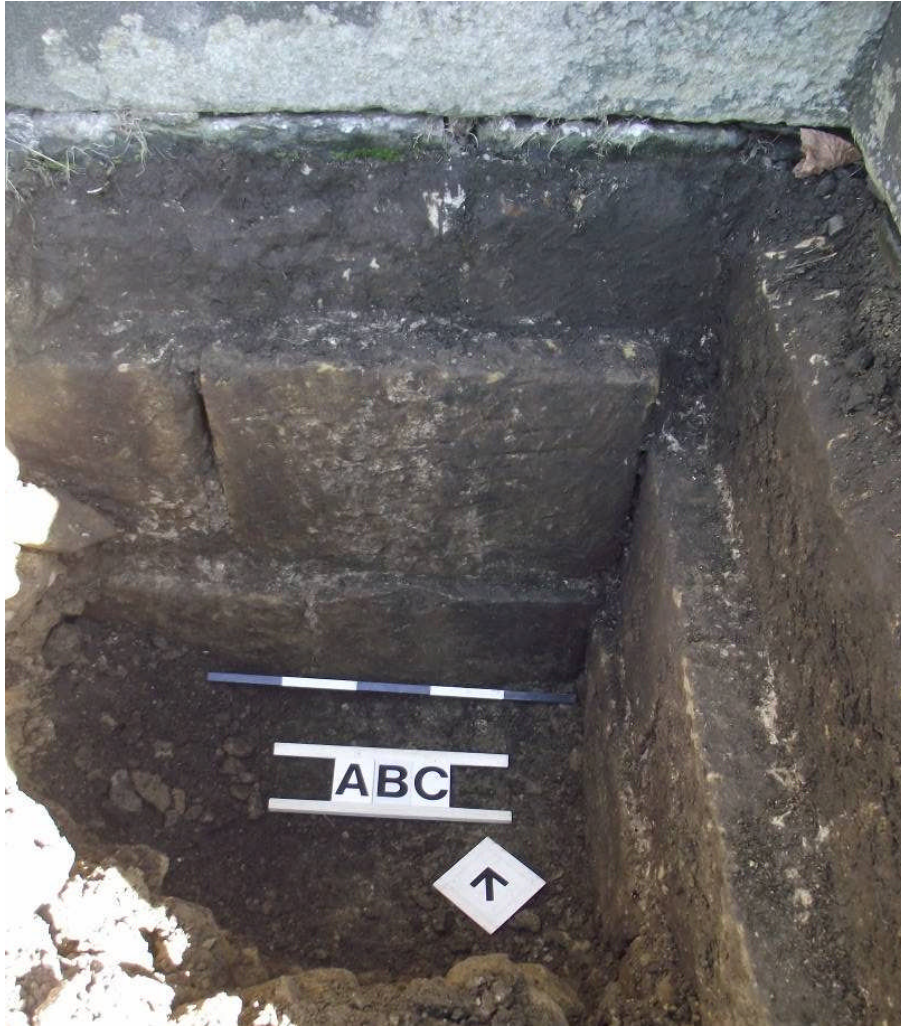
Plate 13: Area 07 showing exposed south transept foundations. Looking north.
