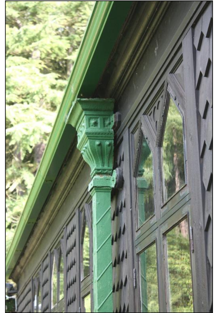
Plate 10: One of two cast-iron down-pipes with decorative rain-heads.
