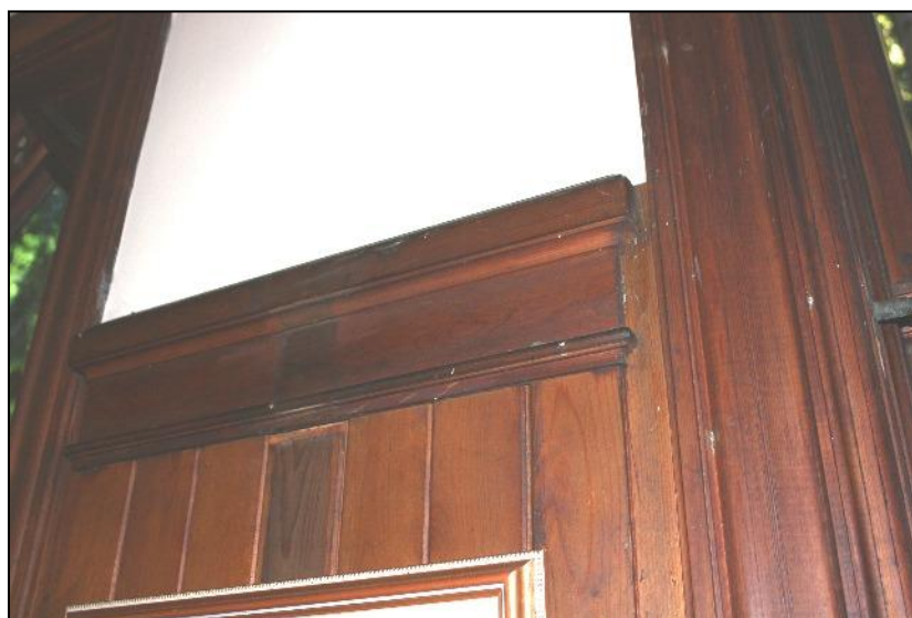
Plate 17: Detail of moulded timbers used inside the chapel.
