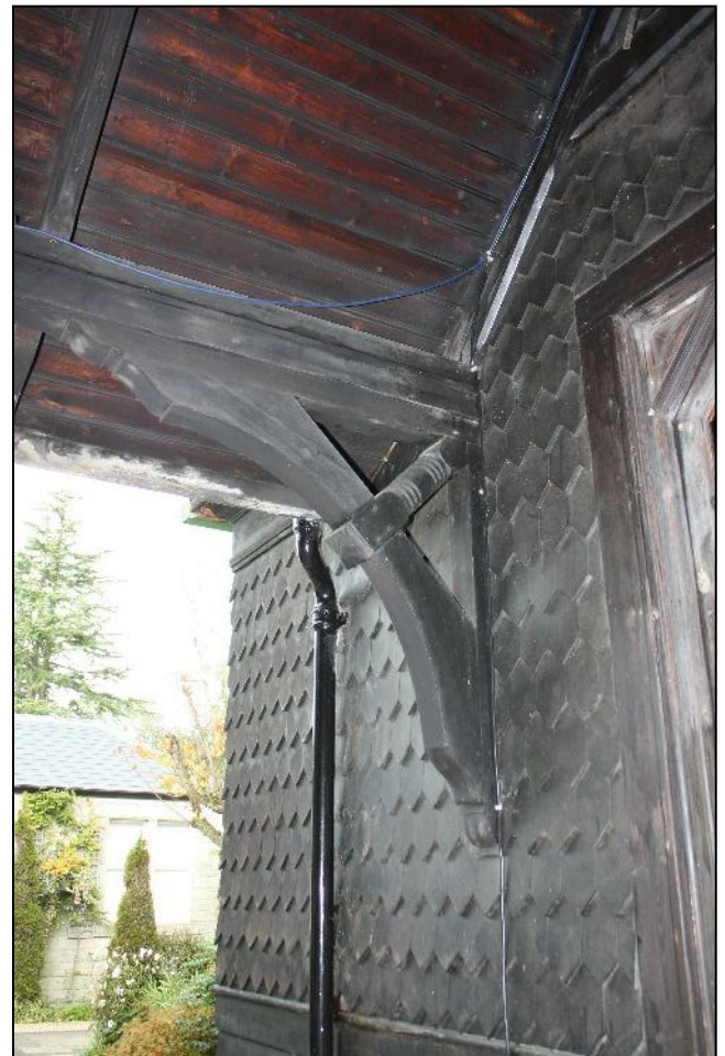
Plate 7: Decorative bracket beneath the walkway canopy.
