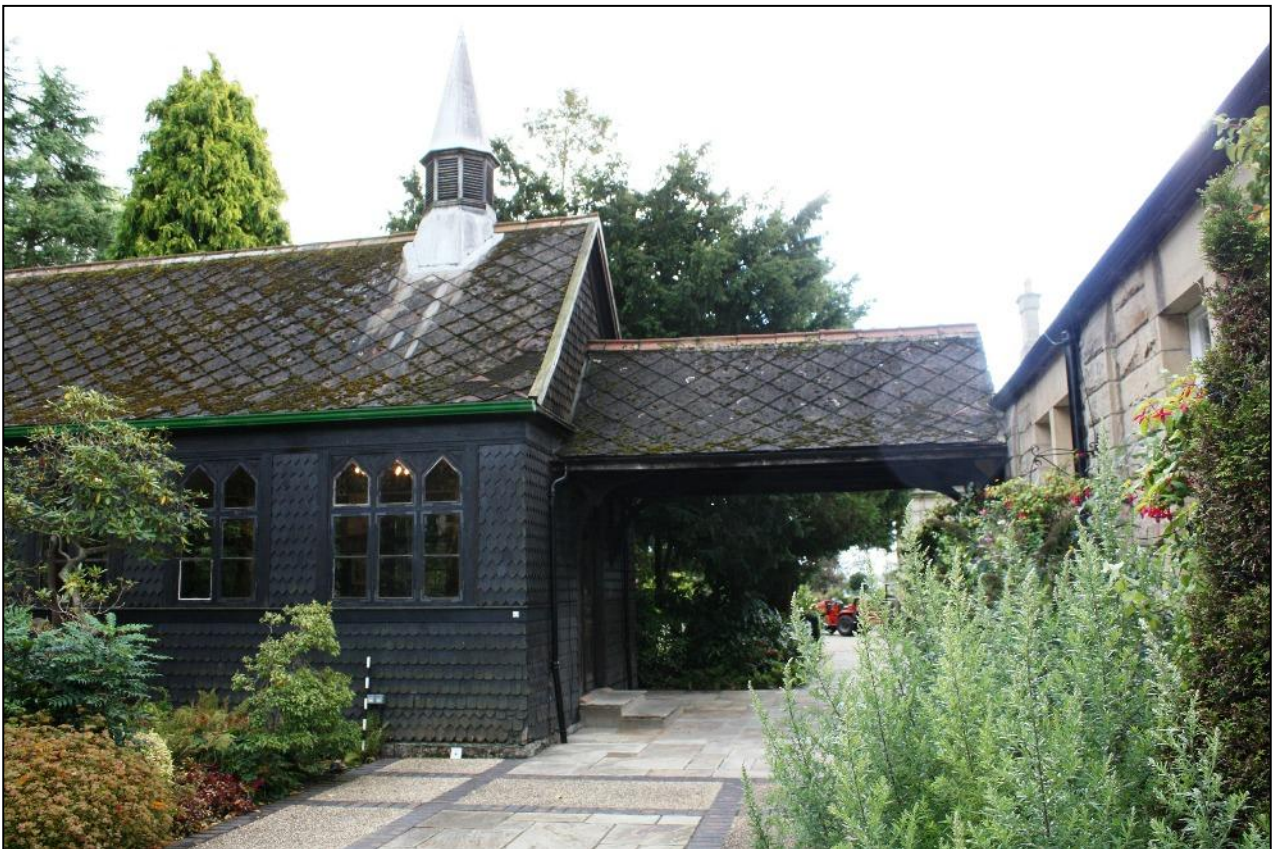
Plate 4: South-west end of the chapel and covered walkway.
