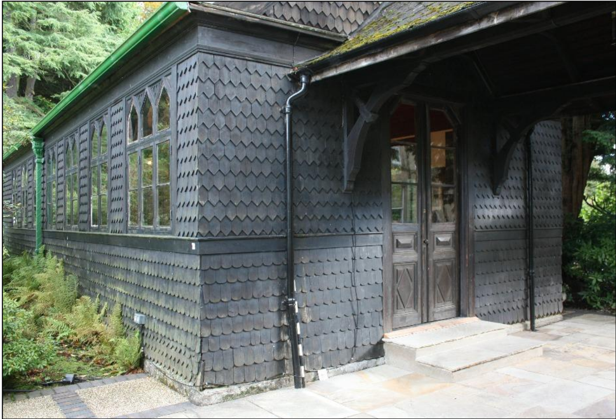
Plate 5: South-west entrance end of the chapel at Stancliffe Hall.
