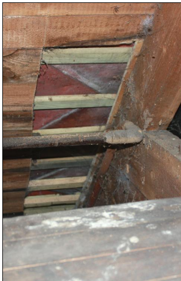
Plate 22: Timber framework showing in the attic beneath asbestos roof-tiles.
