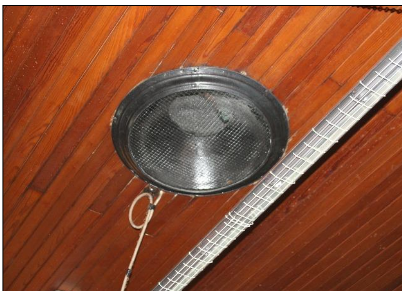
Plate 18: One of the two ventilation openings in the chapel's ceiling.
