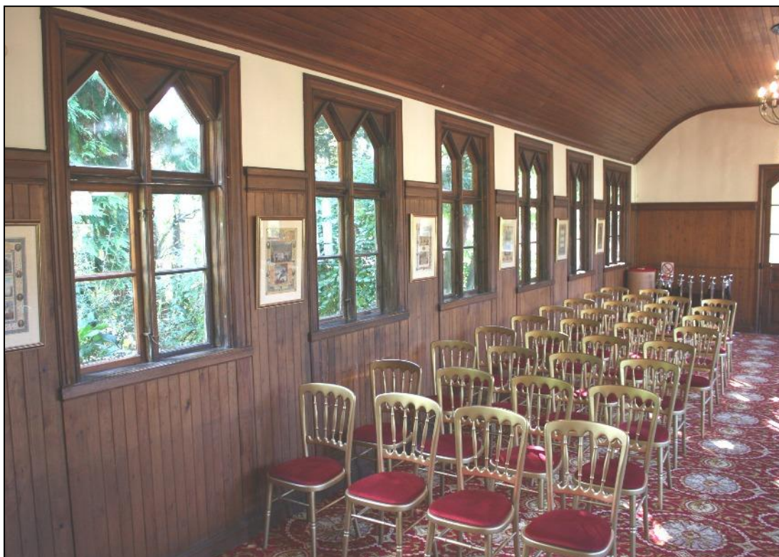
Plate 16: Panelling along one of the internal side walls.
