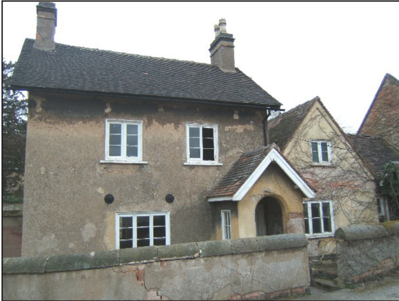
Plate 15: General view of the Cottage with the west extension to the left and the earliest phase of the building to the right, viewed looking north-east
