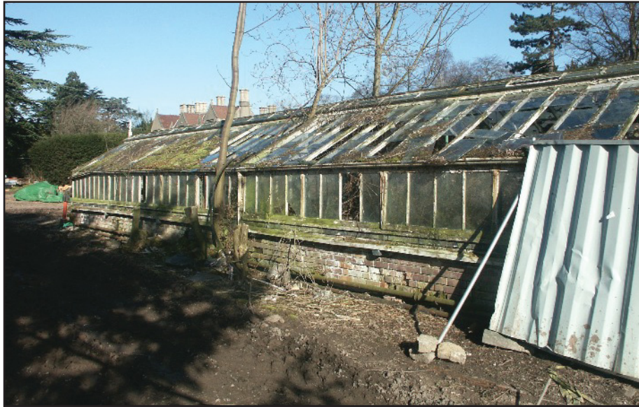
Plate 21: General view of the Hot-house, viewed looking north-west
