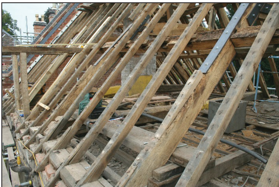
Plate 14: General view of the East Barn's roof, viewed looking north-west
