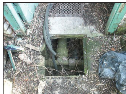
Plate 25: Heating pipe beneath the centre of the Hot-house, viewed looking west
