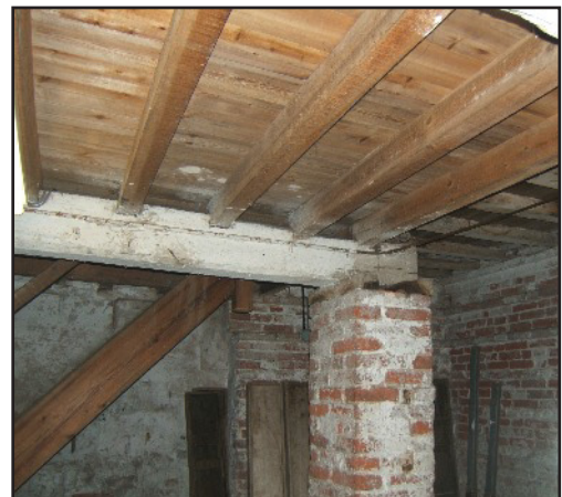
Plate 8: Original brick pier and ceiling beam with later joists, flooring and stair in the Dovecote, viewed looking north-west
