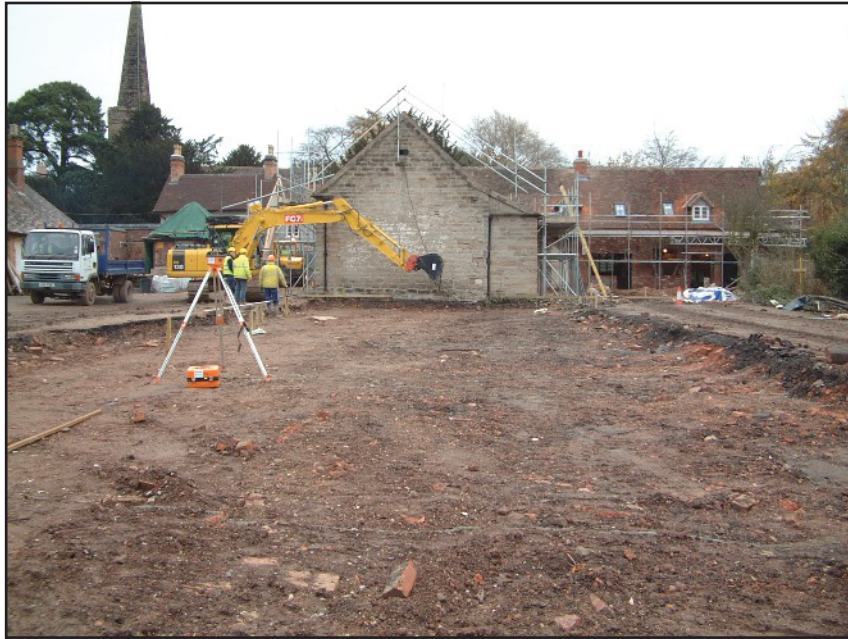
Plate 31: General view of Building Plots 23-30 prior to trenching, viewed looking north-east
