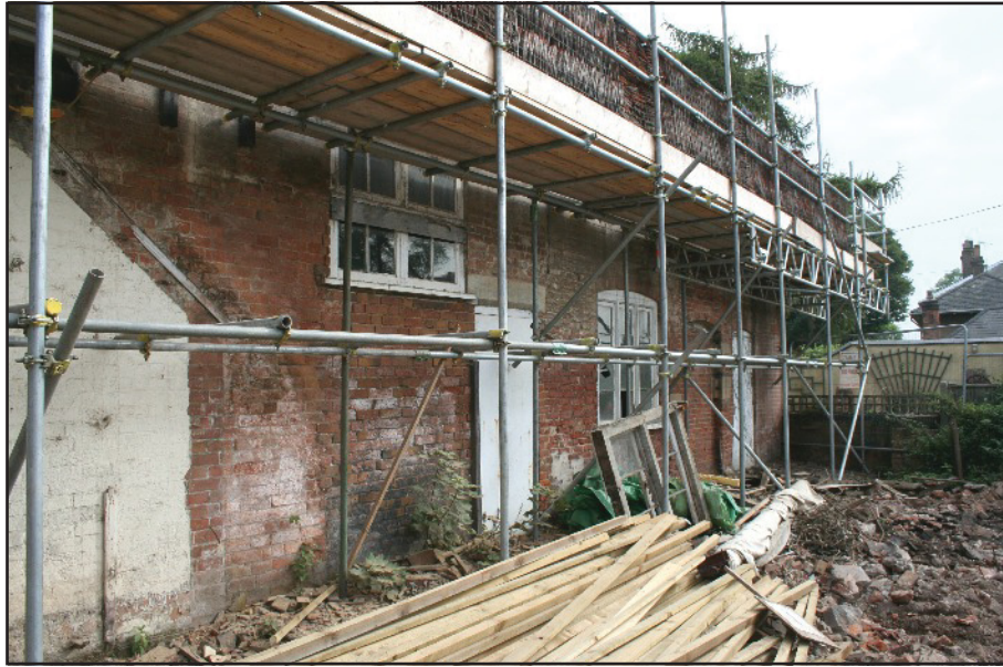
Plate 11: General view of the East Barn, viewed looking north-east
