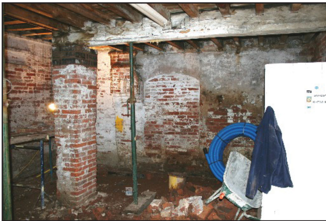
Plate 7: Interior of the Dovecote with the blocked arched doorway on the east elevation in the centre of the picture, viewed looking north-east
