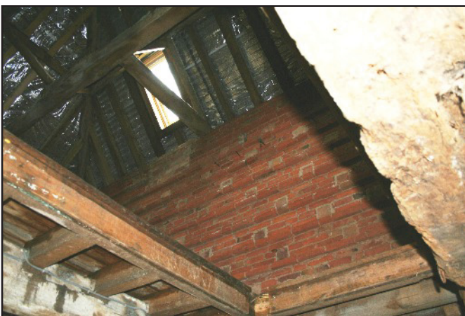
Plate 9: Upper floor nest boxes within the Dovecote, viewed looking south-east
