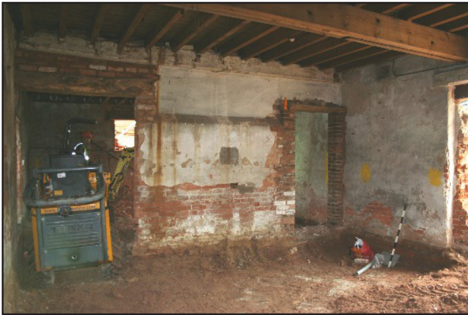
Plate 3: The inserted dividing wall in the West Barn, viewed looking north-east
