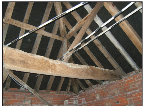
Plate 10: Roof structure of the Dovecote, viewed looking north-east
