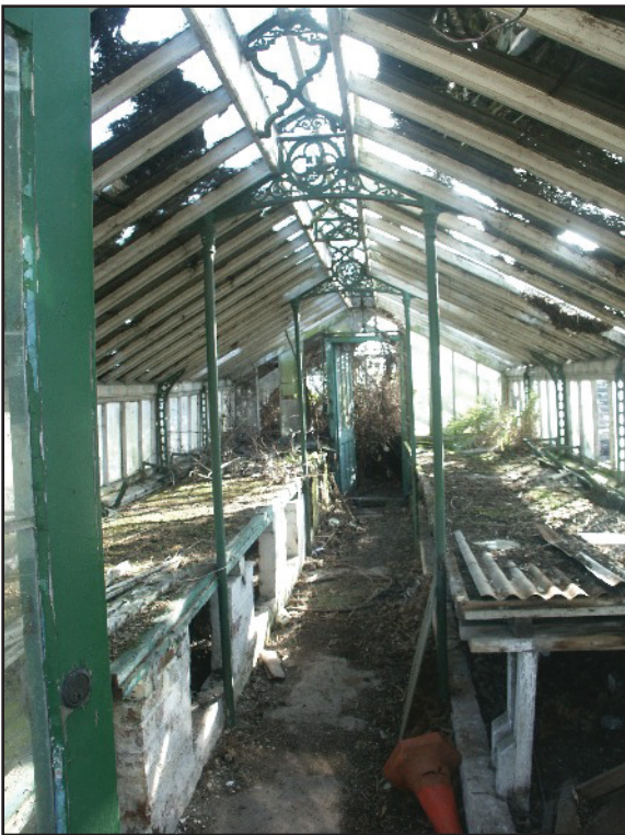
Plate 22: General view of the interior of the Hot-house, viewed looking west
