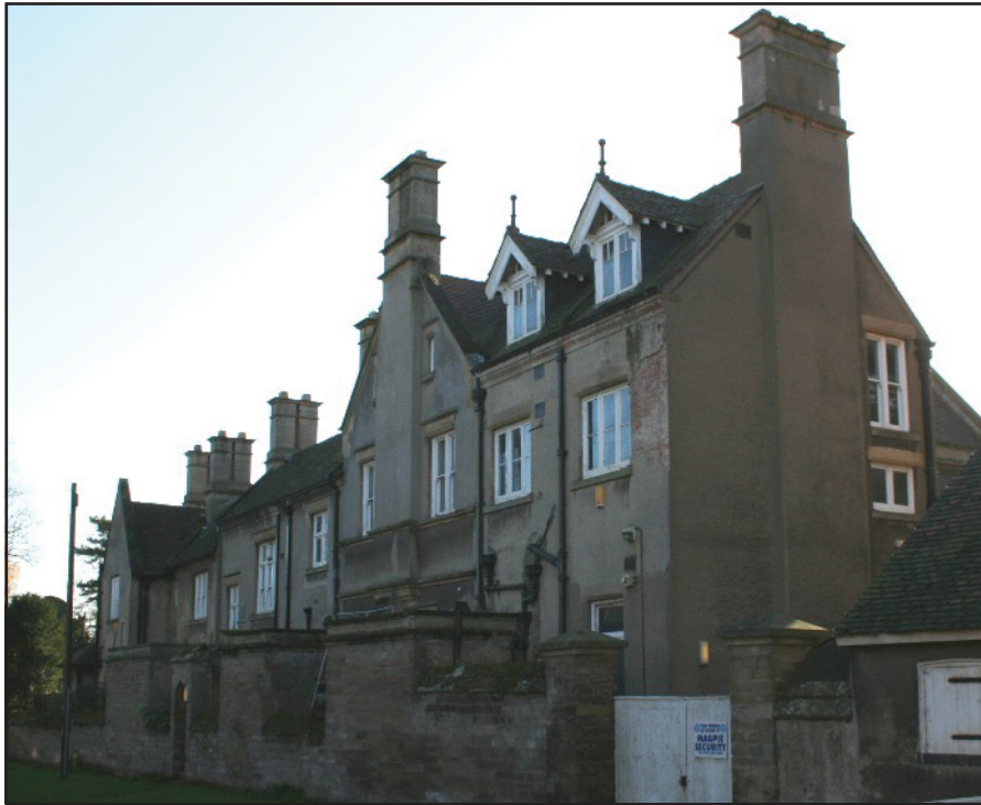
Plate 26: North elevation of Epperstone Manor House, viewed looking south-east
