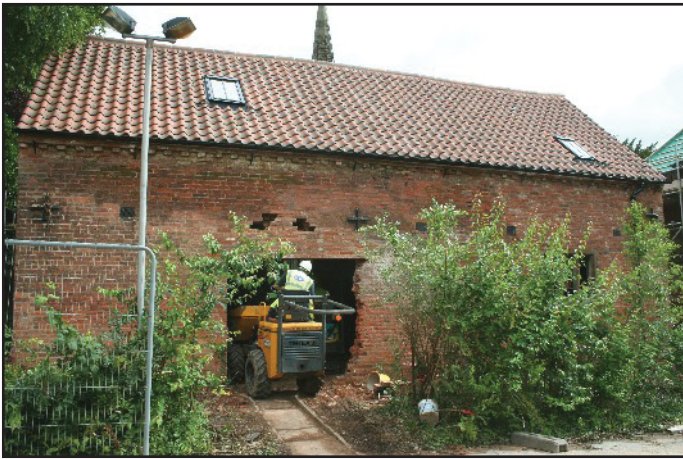
Plate 1: South elevation of the West Barn, viewed looking north-east
