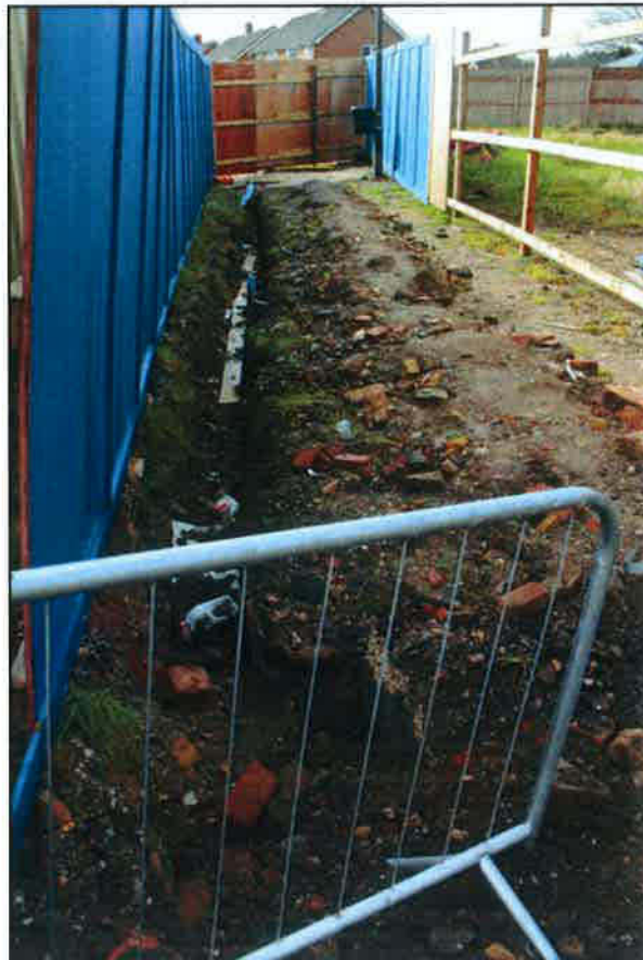
Plate 5: Cable laying in Area B looking west
