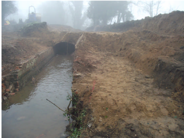
Plate 13. Culvert during demolition from the south west. Looking north east
