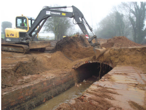
Plate 15. Culvert during demolition. Looking north
