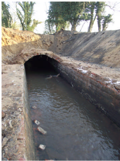
Plate 17. Culvert during demolition. Looking north
