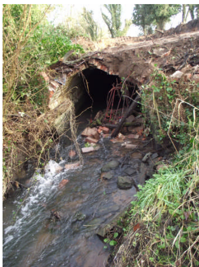
Plate 12. South west end of culvert. Looking north-north east.
