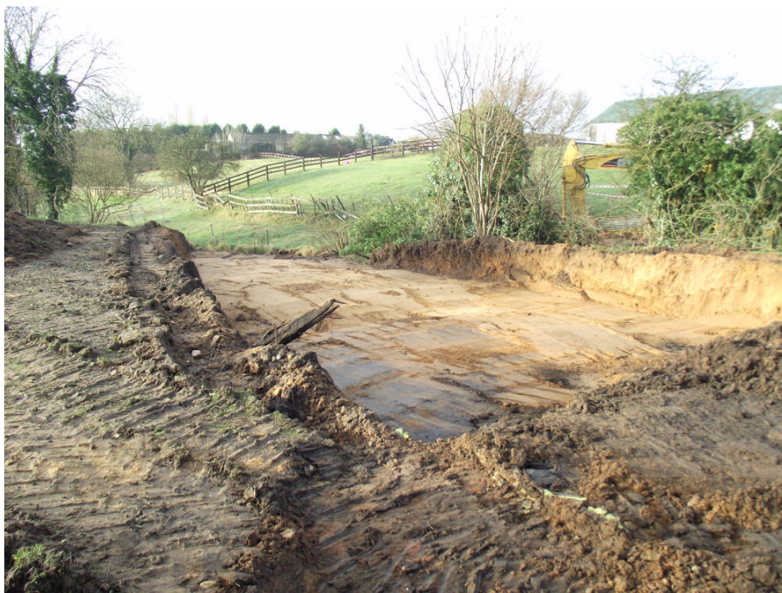
Plate 2. The section the embankment during excavation. Looking north.
