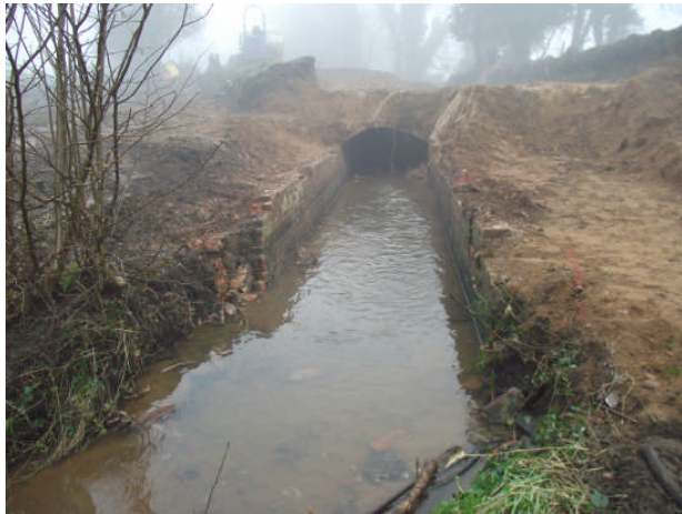
Plate 14. Culvert during demolition from the south west. Looking north east
