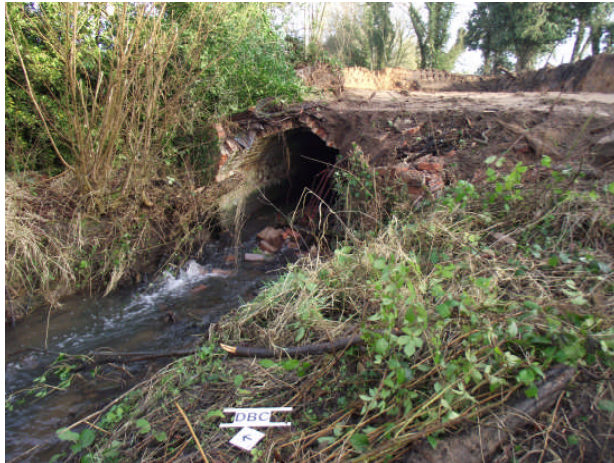
Plate 11. South west end of culvert. Looking north-north east
