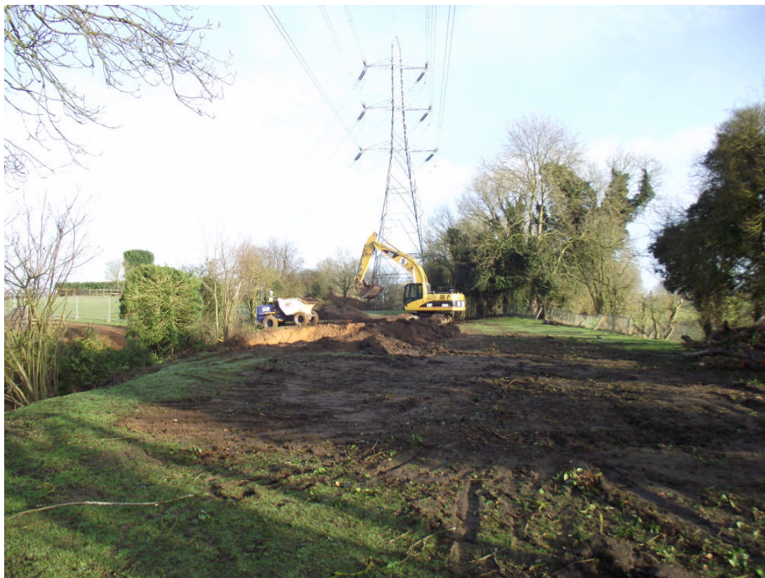
Plate 1. Excavating the section through the embankment. Looking north east.
