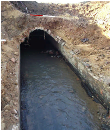
Plate 19. North east end of culvert during demolition. Looking south west
