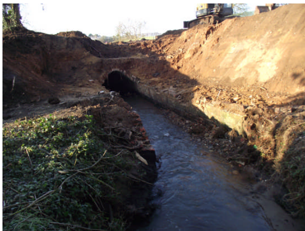
Plate 18. North east end of culvert during demolition. Looking west south west
