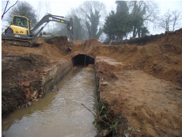
Plate 16. Culvert during demolition Looking north east
