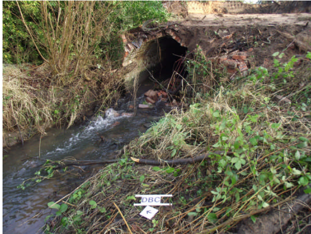
Plate 10. South west end of culvert. Looking north-north east
