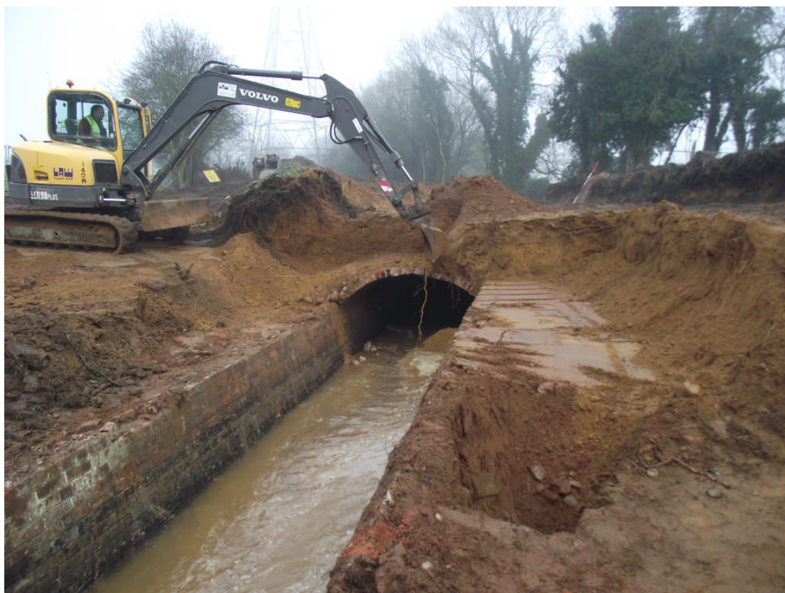
Plate 7. The culvert during demolition. Looking north east.
