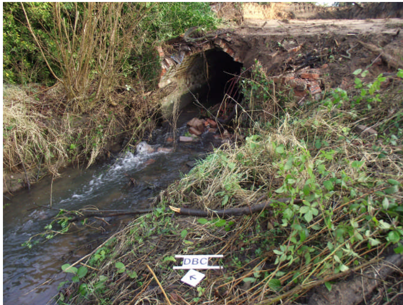
South west end of Dawley Brook Culvert emerging from the embankment.
