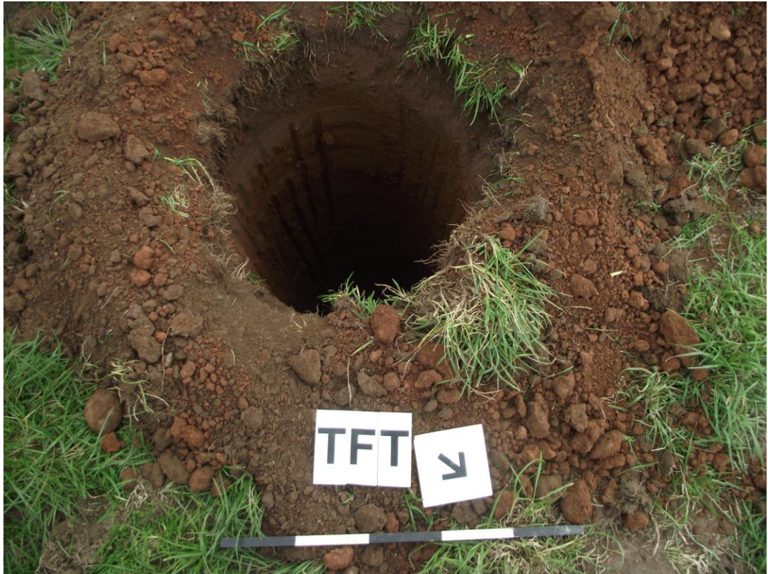
Plate 9. area 04 on completion of augering. Looking south west.
