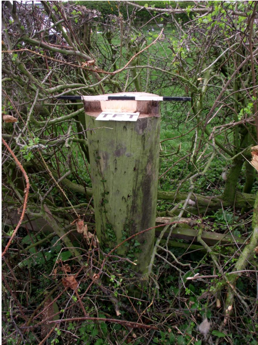
Plate 11. Redundant cable pole cut to the level of the hedge and left in situ . Looking south.
