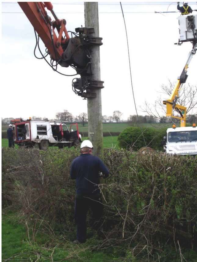
Plate 10. Removing redundant cable pole. Looking south west.
