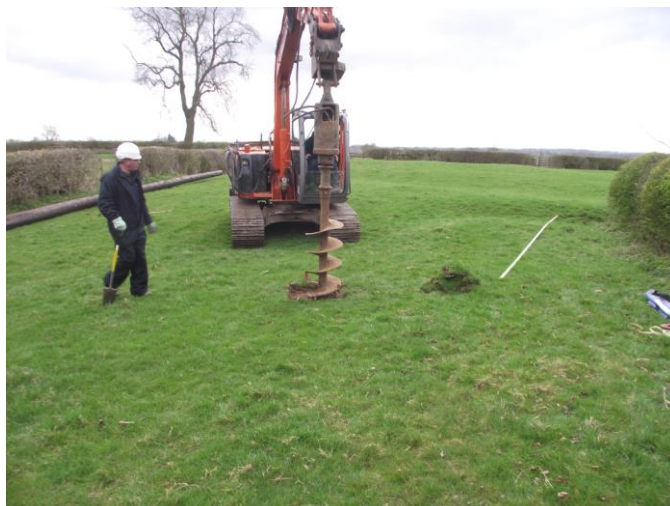
Augering in the Scheduled Area of Thurvaston Farm.
