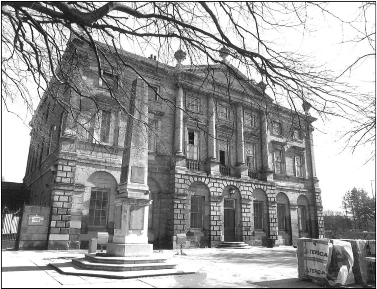
Plate 1: West elevation of St. Helen's House, viewed looking south-east.
