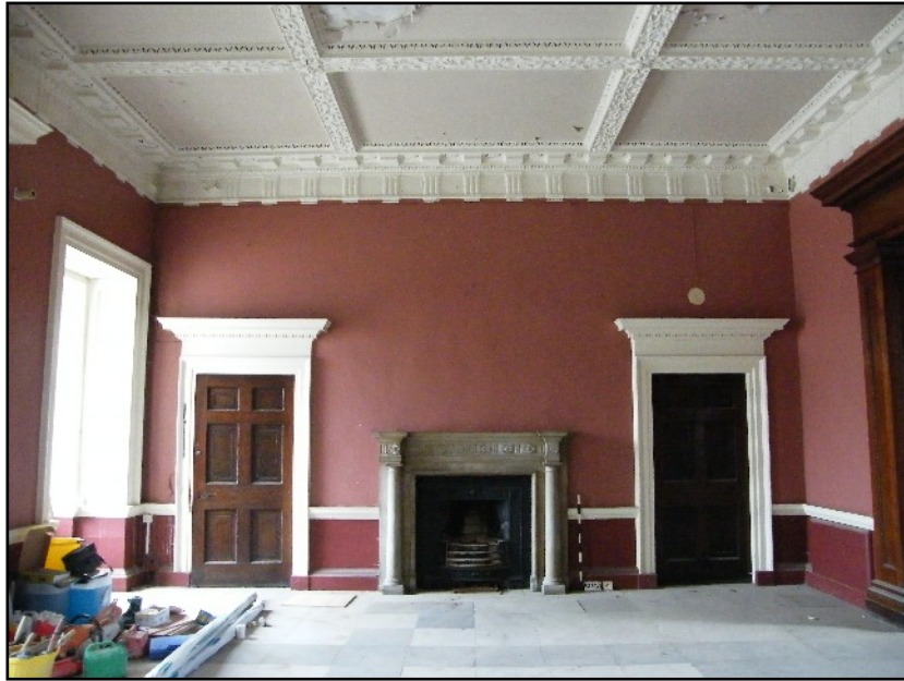
Plate 3: North wall of room SHG1, viewed looking north.
