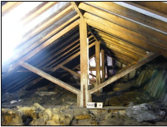
Plate 23: Roof over room SH29, viewed looking west.
