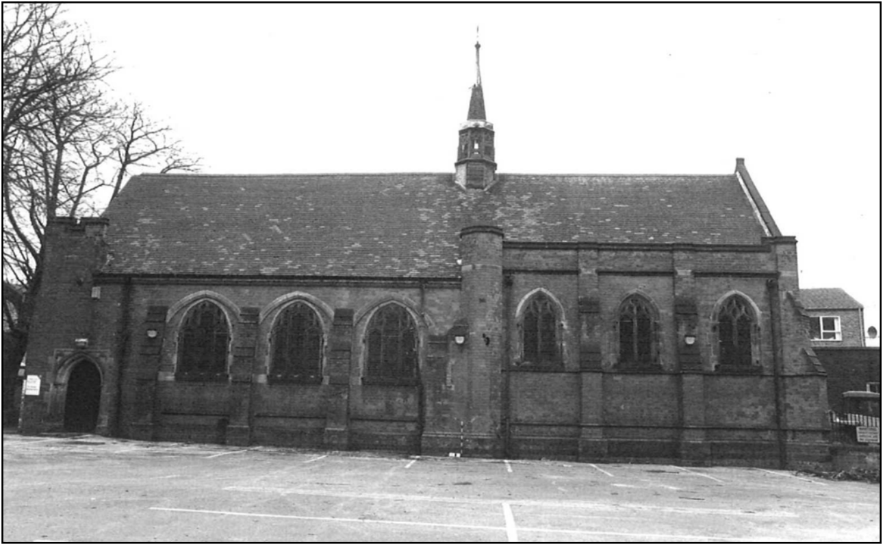
Plate 29: South elevation of the Chapel, viewed looking north.
