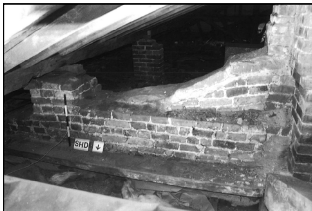
Plate 25: Northern face of the early external wall with the finial base to the east and chimney to the west, viewed looking south-east.
