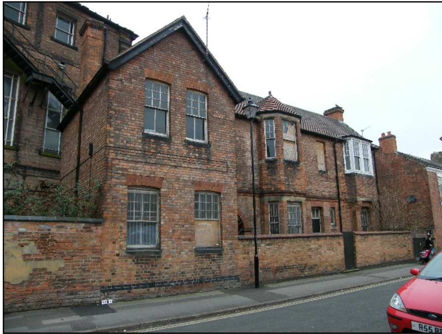
Plate 31: The east elevation of the Headmasters House, viewed looking north-west.
