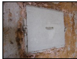
Plate 19: Metal hatch in the north wall of SH27, viewed looking north-east.
