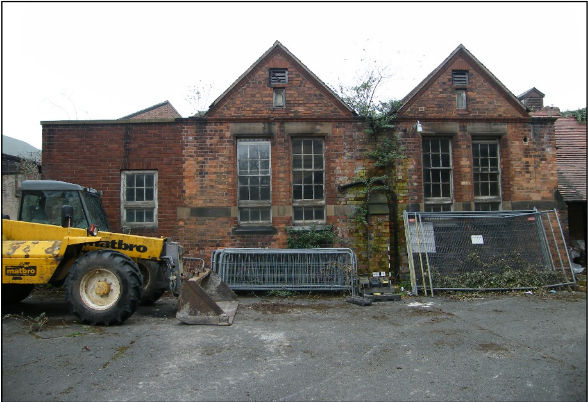
Plate 36: The south elevation of the Chemistry Laboratory, viewed looking north.
