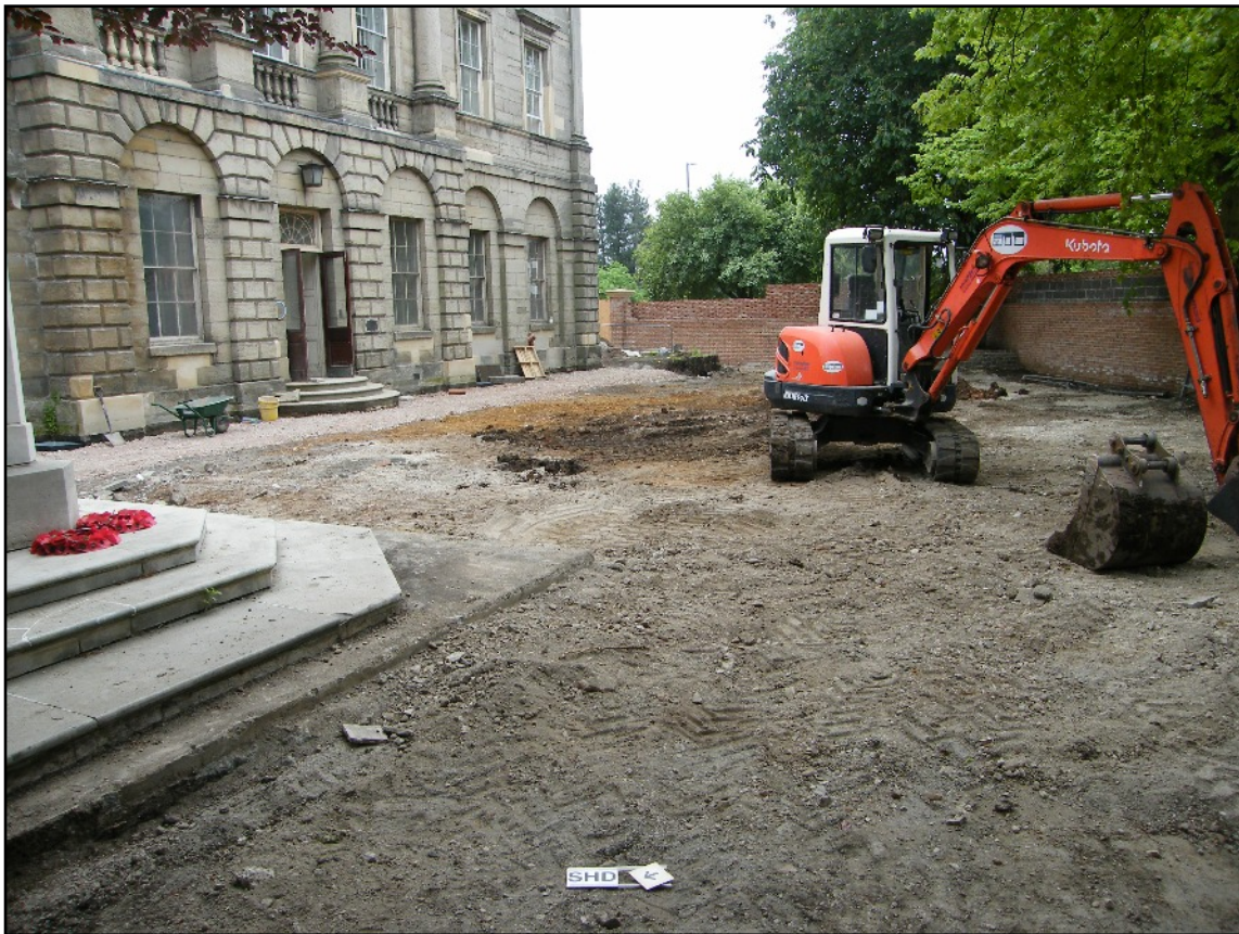
Plate 39: Machine stripping in Area 01, viewed looking south-east.
