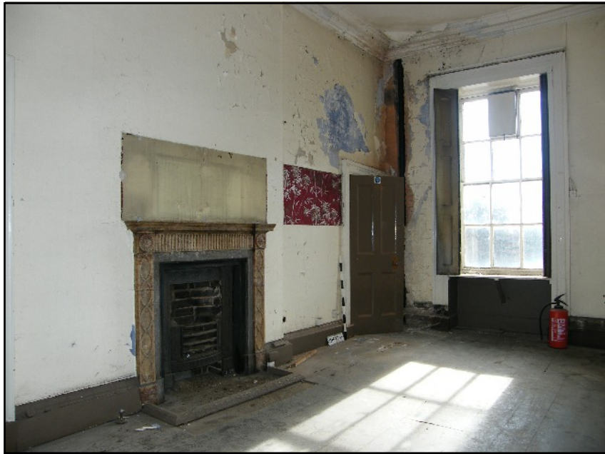
Plate 12: General view of room SHF15, viewed looking south-east.
