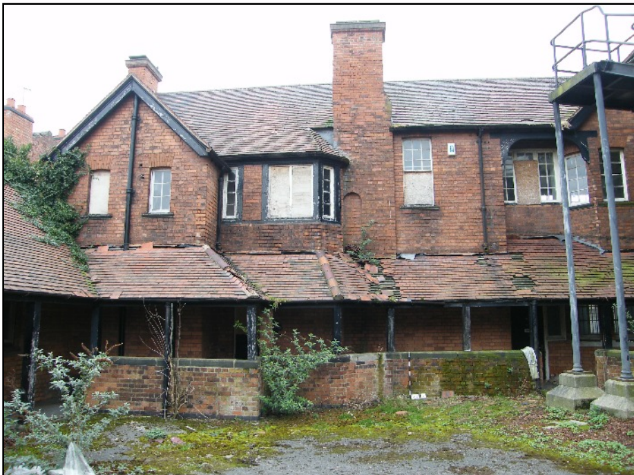
Plate 32: The west elevation of the Headmasters House, viewed looking west.
