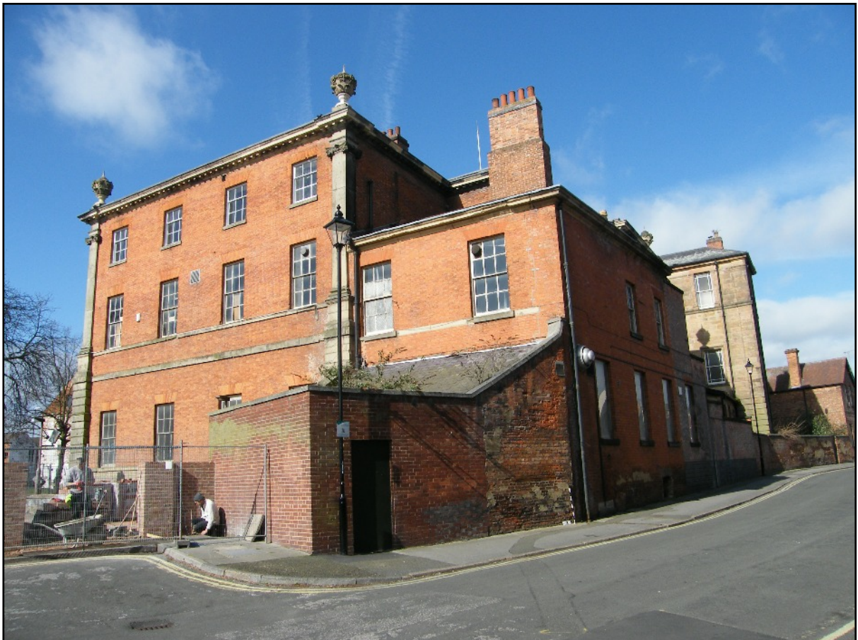
Plate 2: South elevation of St. Helen's House, viewed looking north-west.
