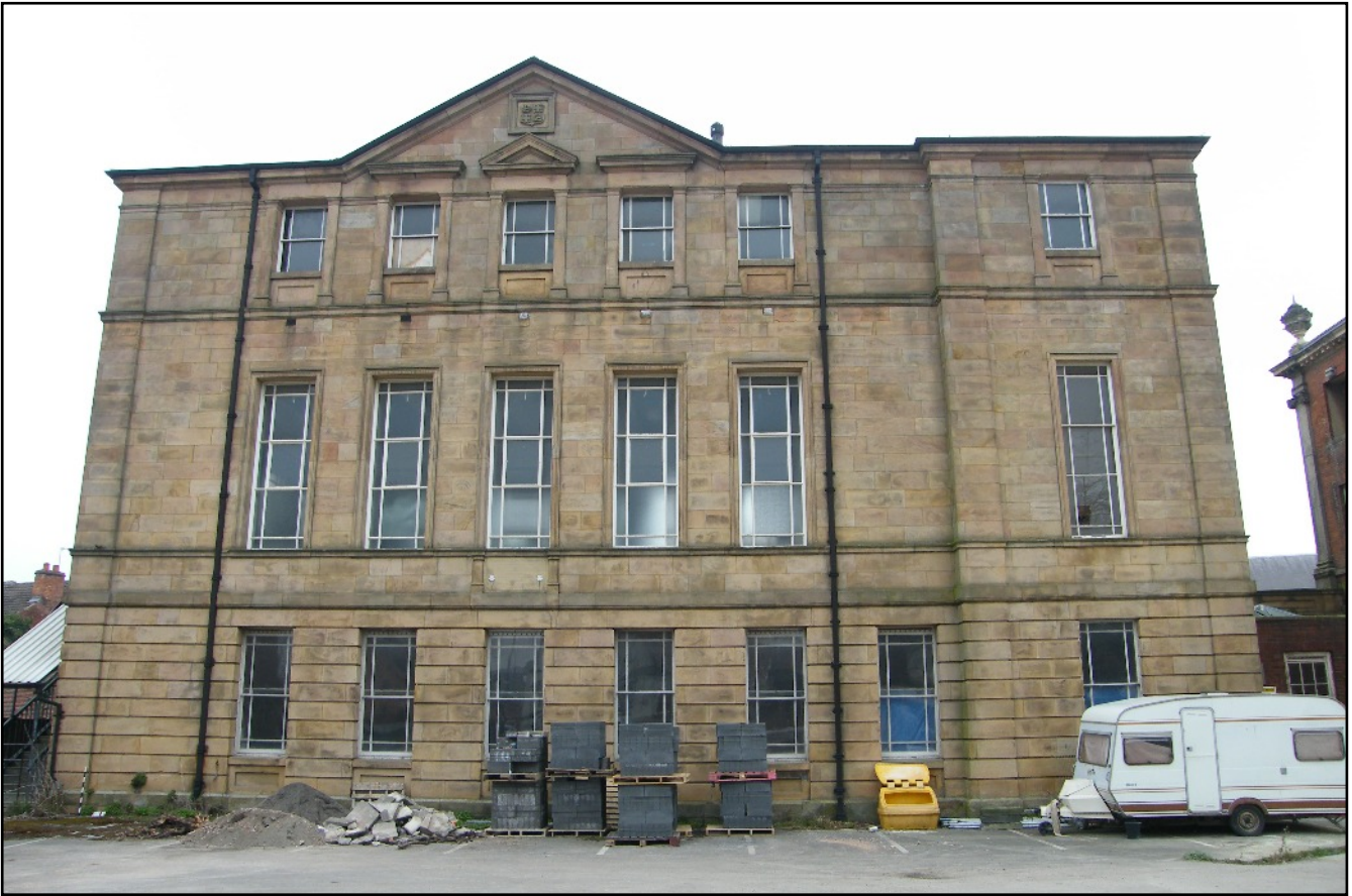
Plate 27: West elevation of the Pearson Building, viewed looking east.
