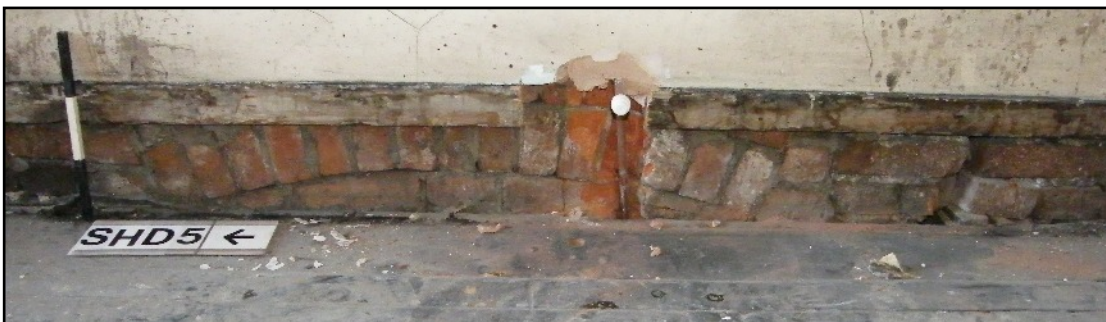
Plate 16: The brick arch in room SHF5, viewed looking east.
