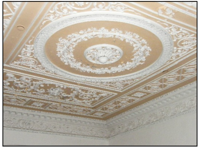
Plate 5: Detail of the plaster ceiling of room SHG3, viewed looking south-west.
