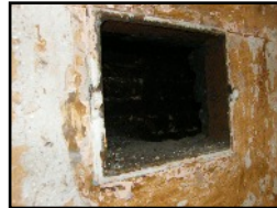
Plate 20: Metal hatch in the north wall of SH27, viewed looking north-east.
