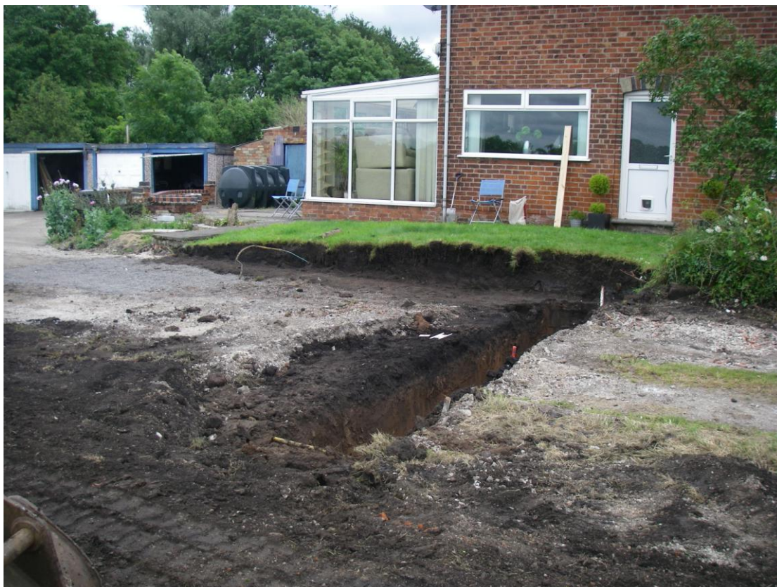
Plate 11 View showing modern garage structures prior to demolition
