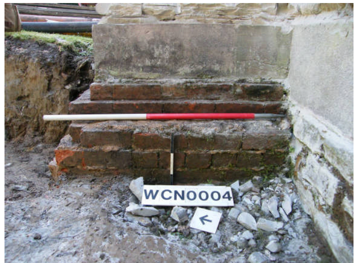
Plate 6: Area 01 looking south (left) and east (right), showing brick buttress foundation 0004.
