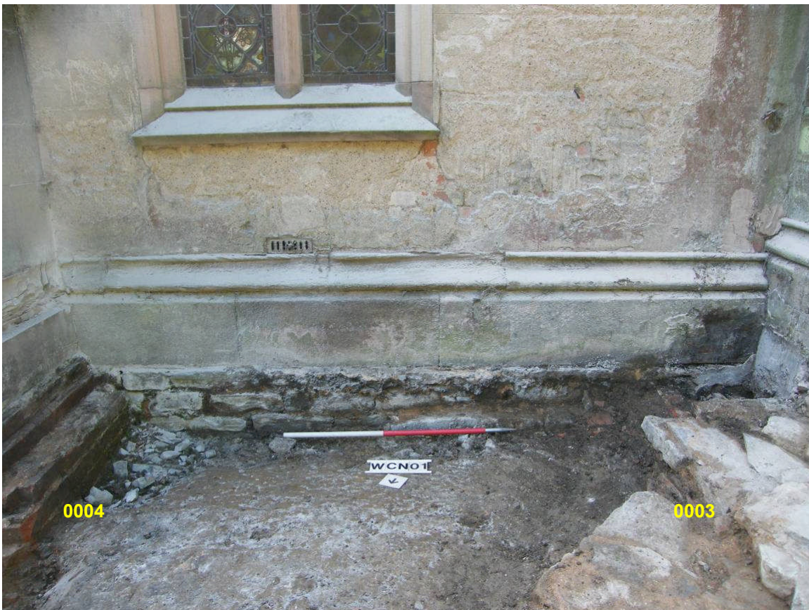
Plate 2: Area 01 looking south, showing brick buttress foundation 0004, stone diagonal tower buttress 0003 and the stone foundations of the north aisle.
