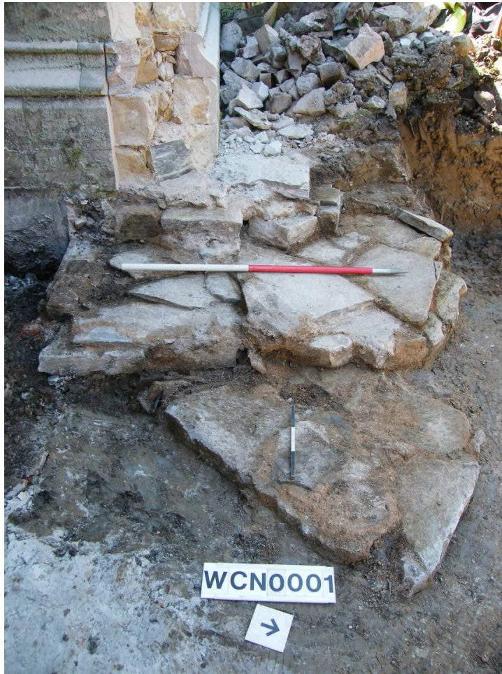
Plate 5: Area 01 looking west, showing stone diagonal tower buttress 0003.
