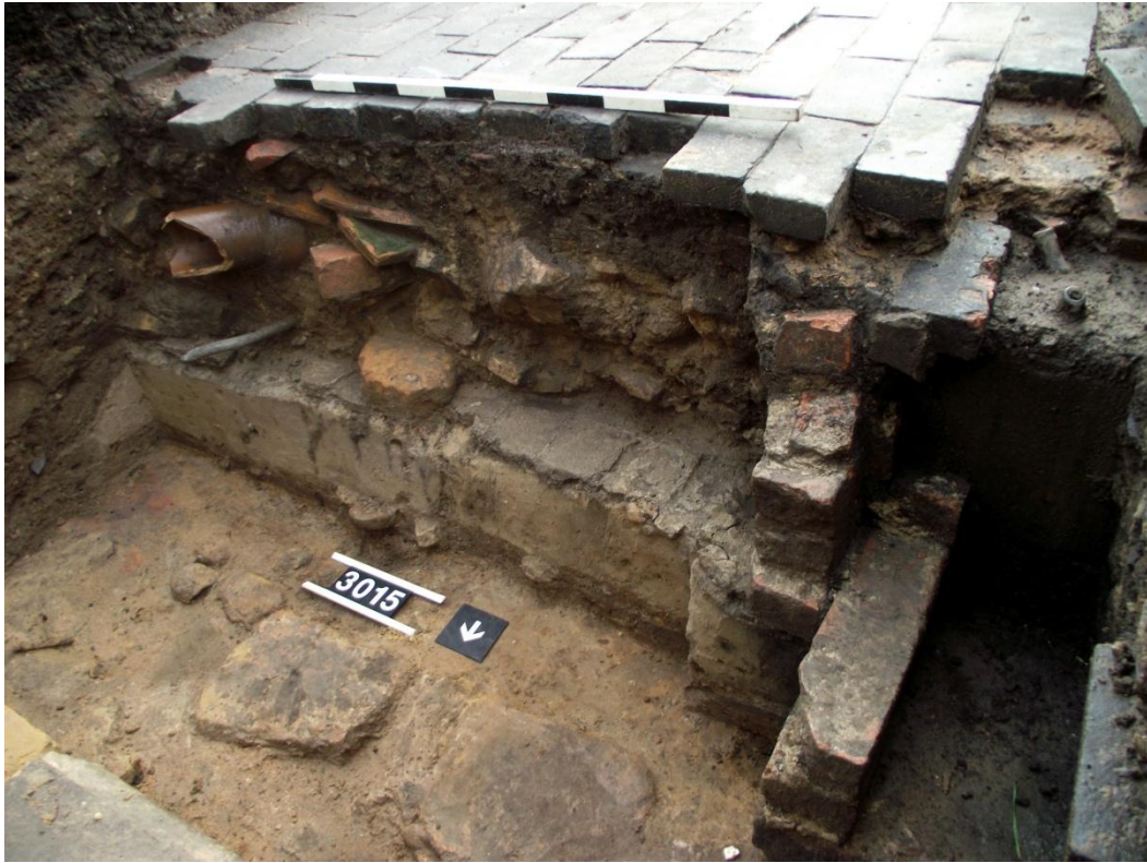
Plate 101: Detail of Trench 3 looking south showing remnant flagged floor of priory church in foreground.
