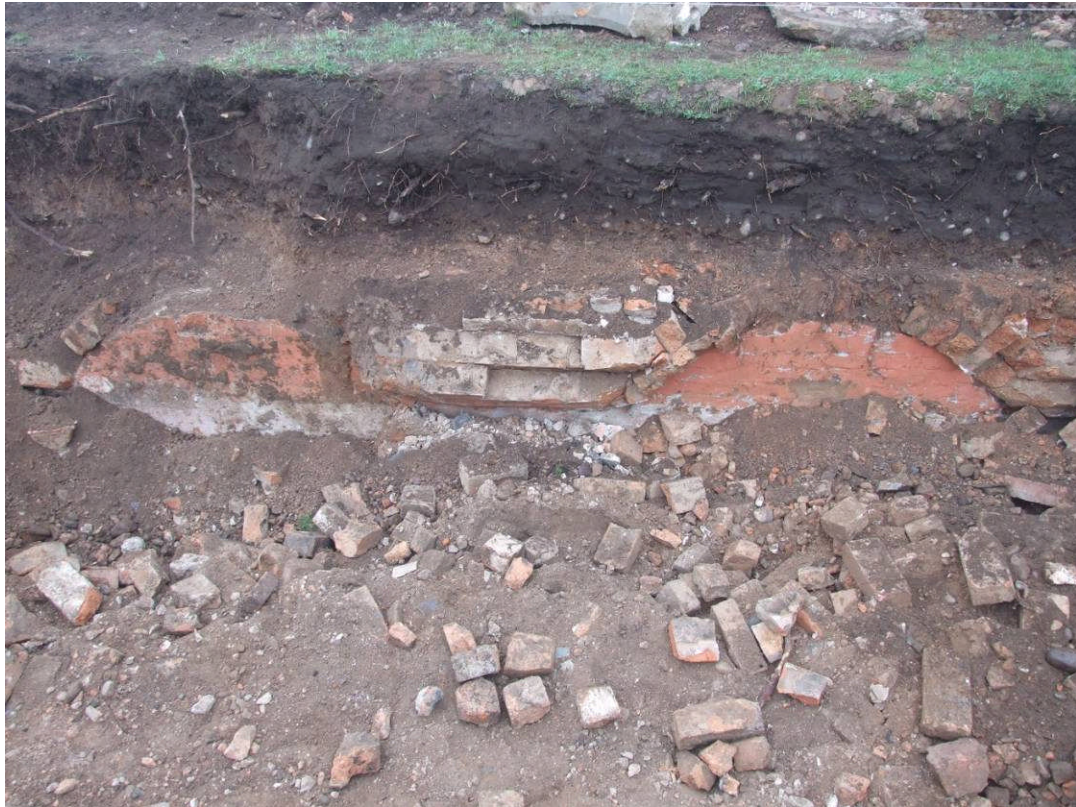
Plate 13: Area 02. Vaulted cellars in the old vicarage with redeposited sand and rubble below topsoil
