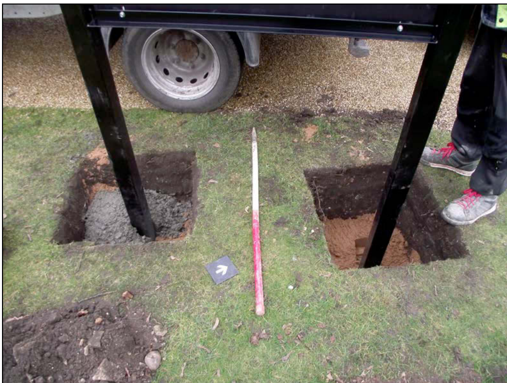
Plate 5. Installation of sign
