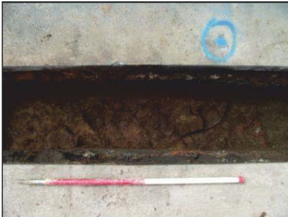
Plate 2. East facing photograph of Wall (0018) and features [0014] [0012]
