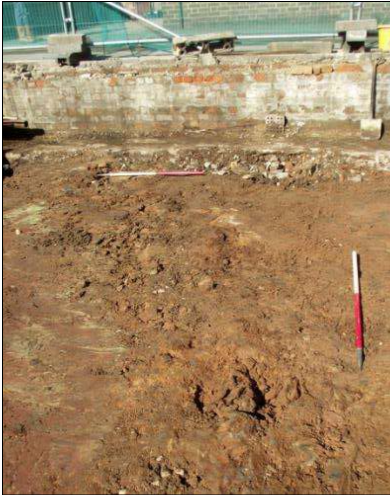
Plate 8. East facing photograph of wall [0024]
