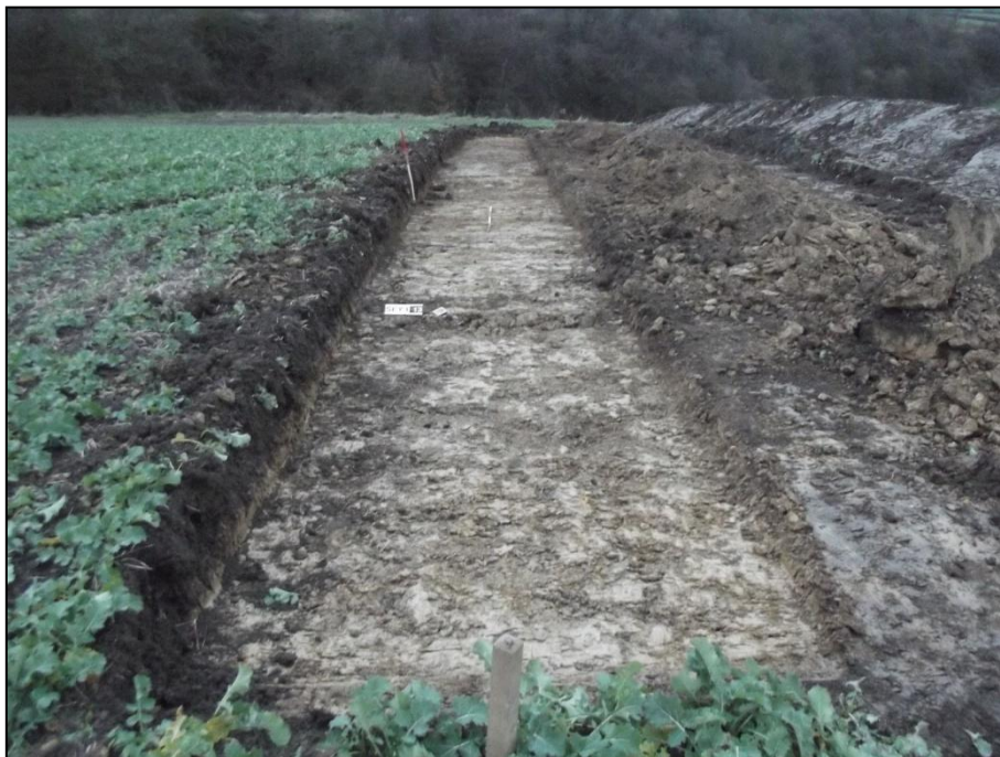
Plate 7: Trench 13 looking NNW
