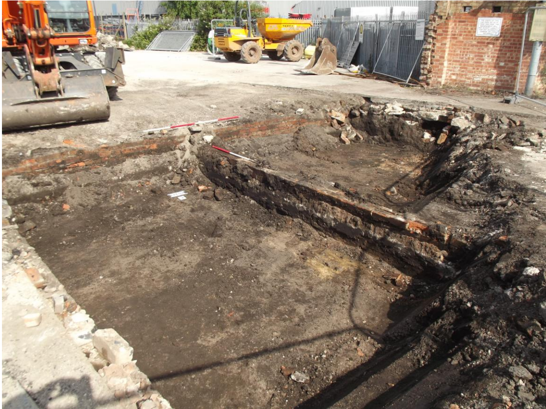
Plate 5: LPE Trench 02, 20th century foundations
