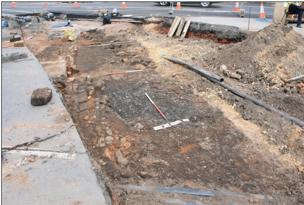
Ground reduction of trackbed in Gregory Street Central (looking W)
