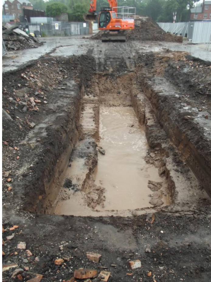
Plate 1: Excavation of Trench 05, looking east.
