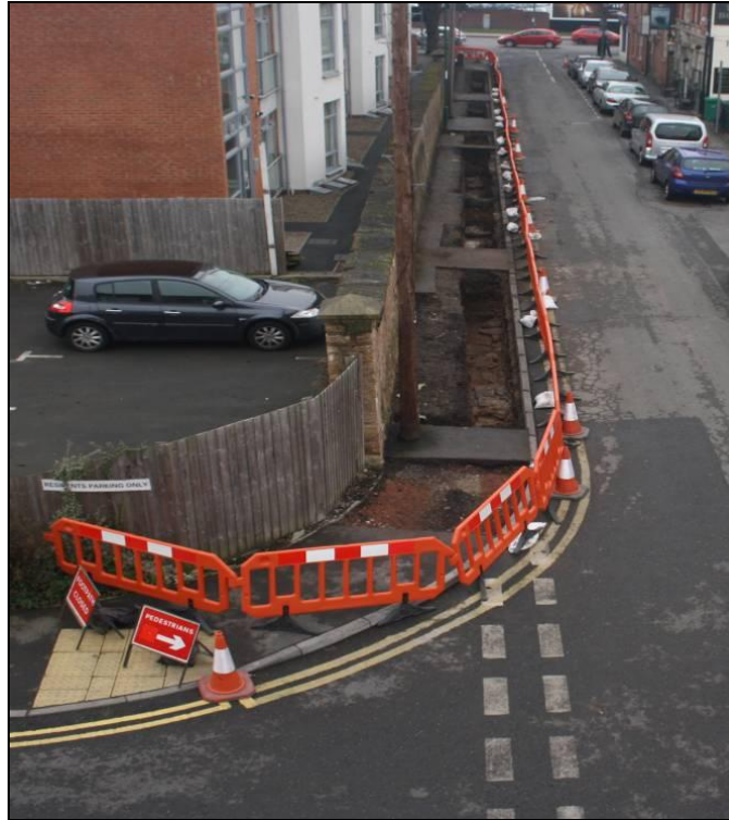
East facing photograph of Trenches 2 through to 10 on Priory Street
