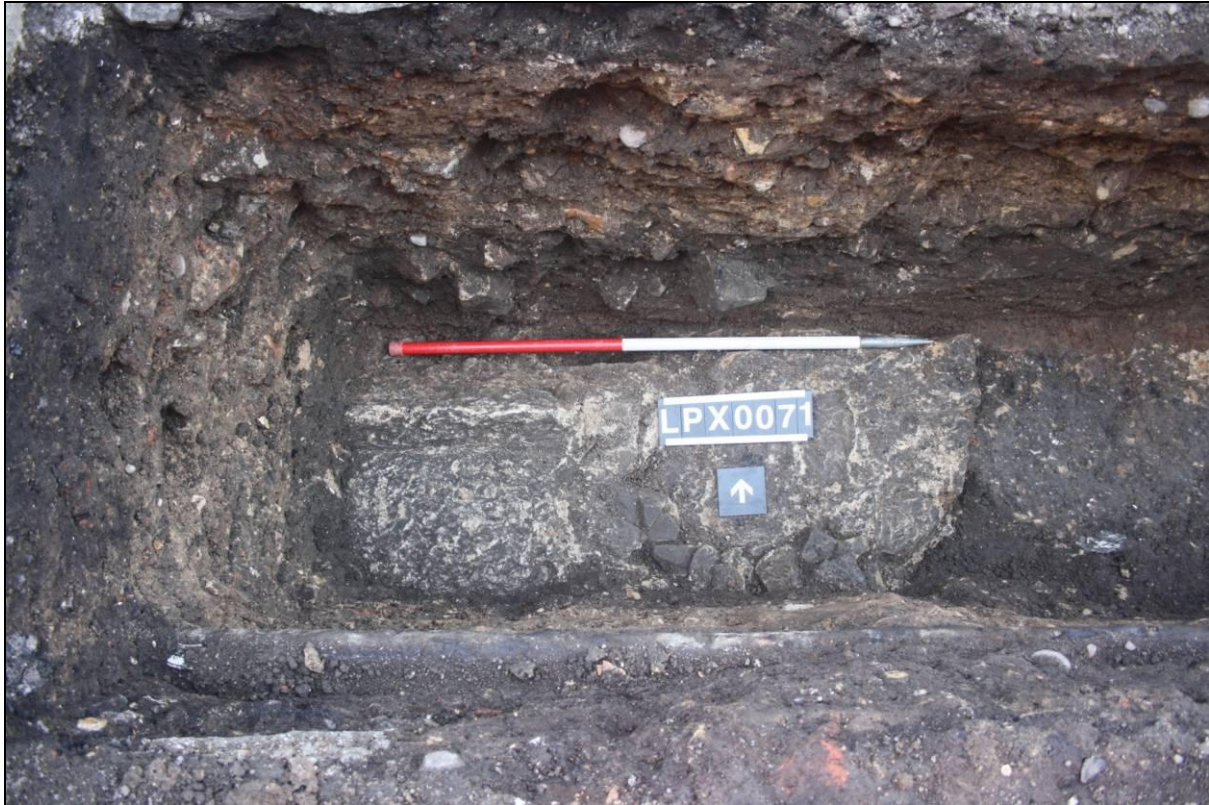
Plate 4. Trench 4, showing lipping in mortar on top of wall 0071 (North to top of photo, 2m scale).
