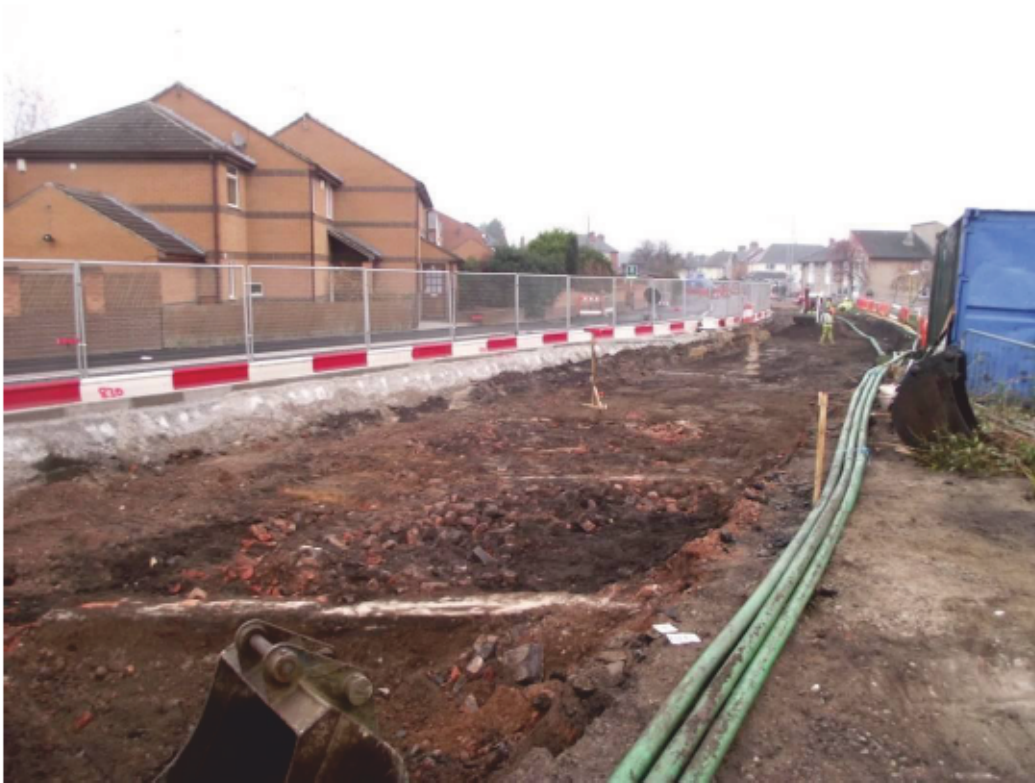
Plate 33. Foundations of possible pub cellar walls (2221) and (2225), looking north-east
