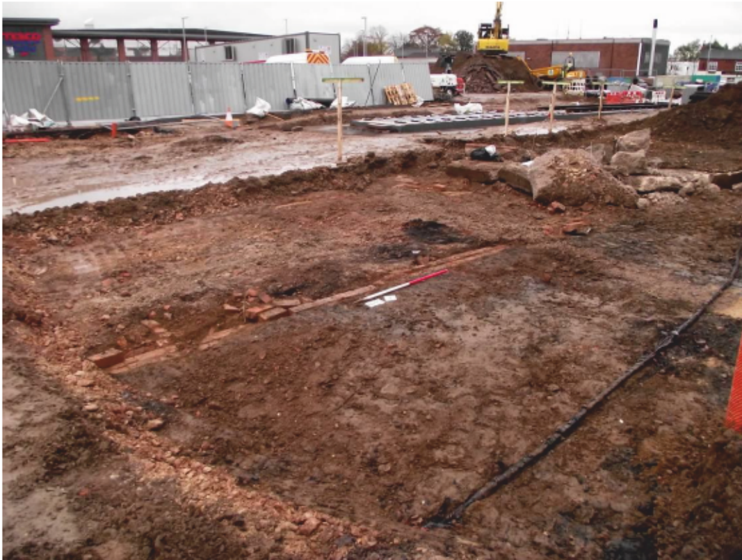
Plate 19. Showing foundations of structure (2142), looking south-east
