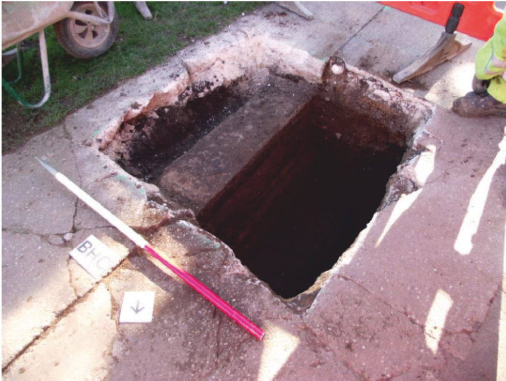
Plate 5. Wall foundation (2407), looking south
