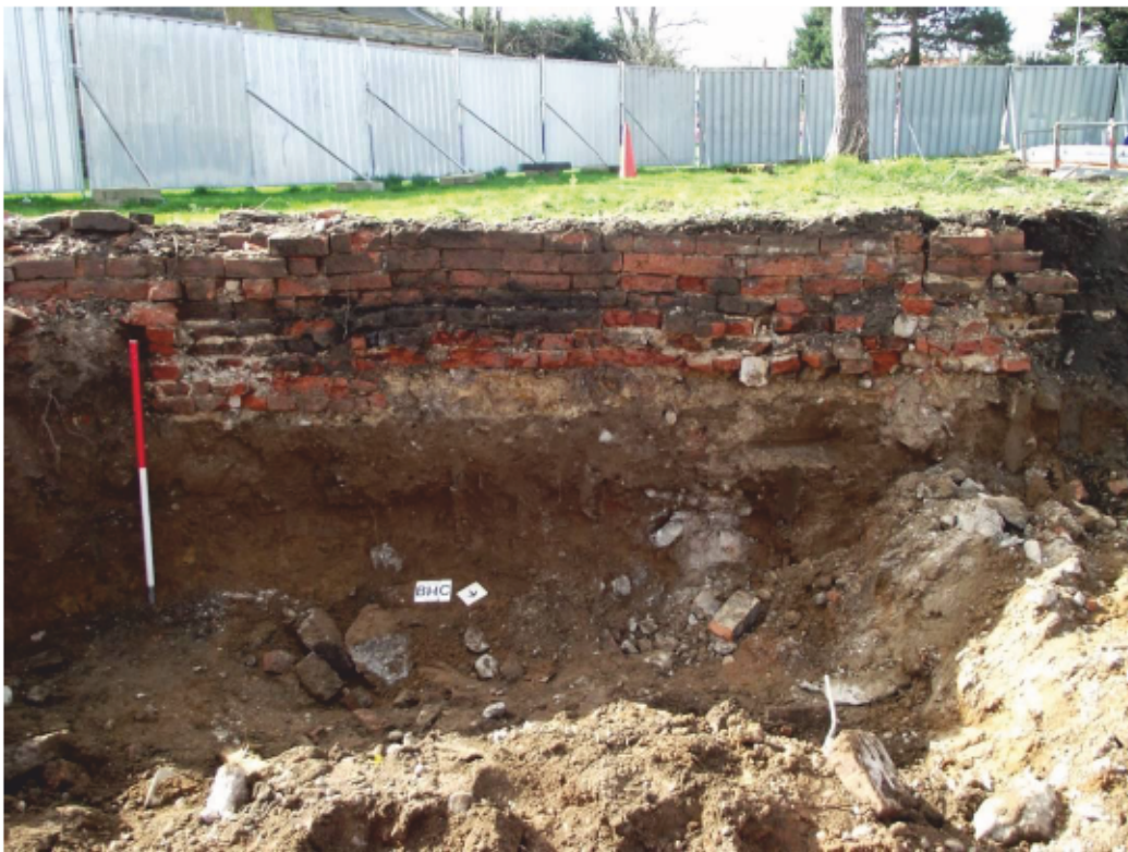
Plate 6. Churchyard walls (0043) and (0044), looking south-west
