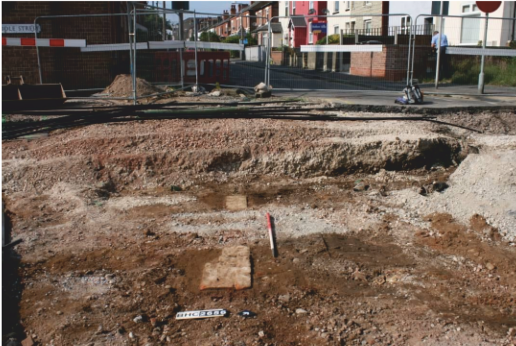
Plate 27. Middle Street foundations (2656), looking north-west
