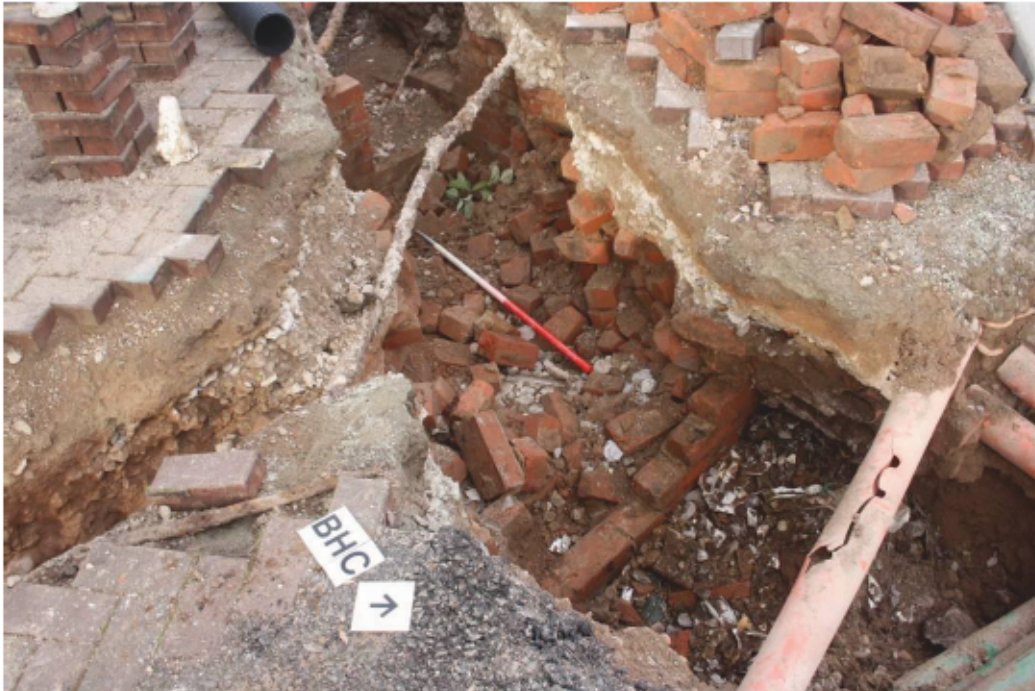
Plate 26. Part of cellar wall foundations (3001), looking west
