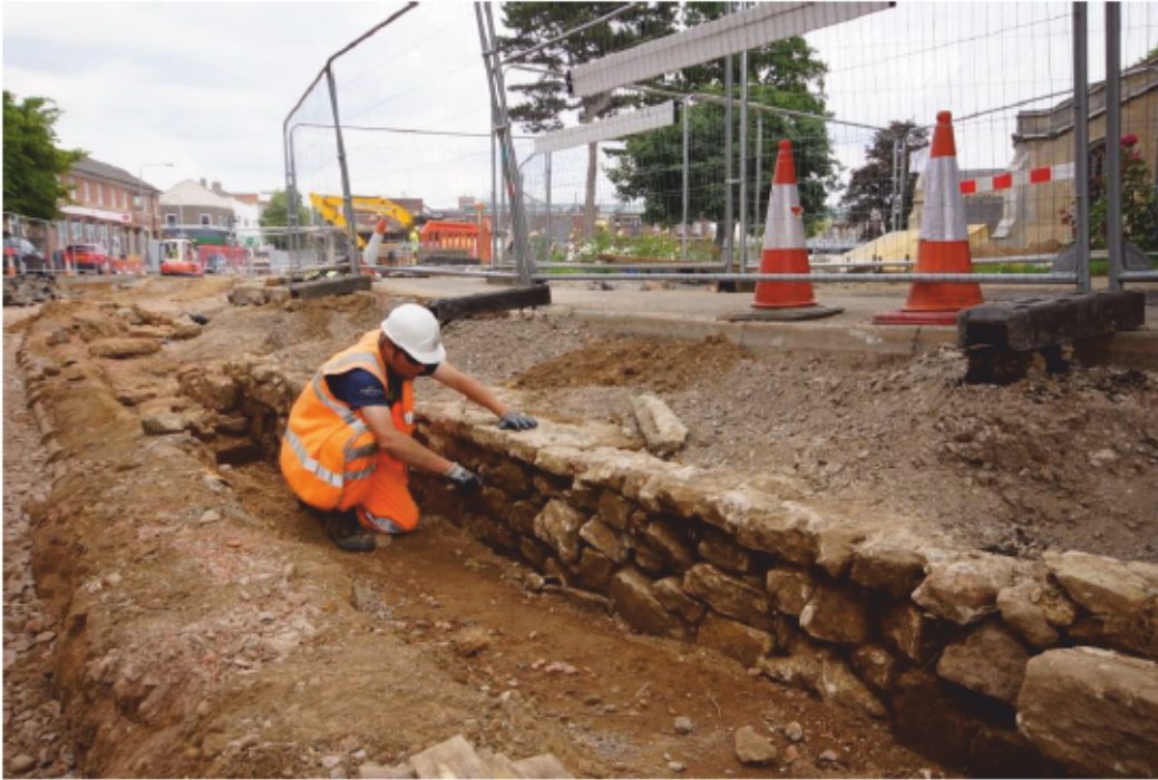
Plate 1. Churchyard wall (2532), looking north-east
