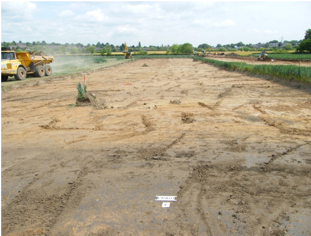
Plate 1: Looking East across the partially-stripped attenuation pond area
