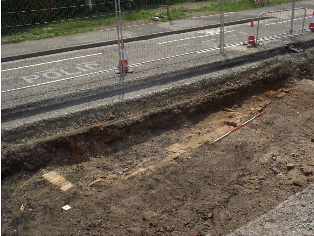
Plate 21: Meadows Way: Plan view of walls (MWN0063), (MWN0064) and (MWN0065). Looking Southeast.
