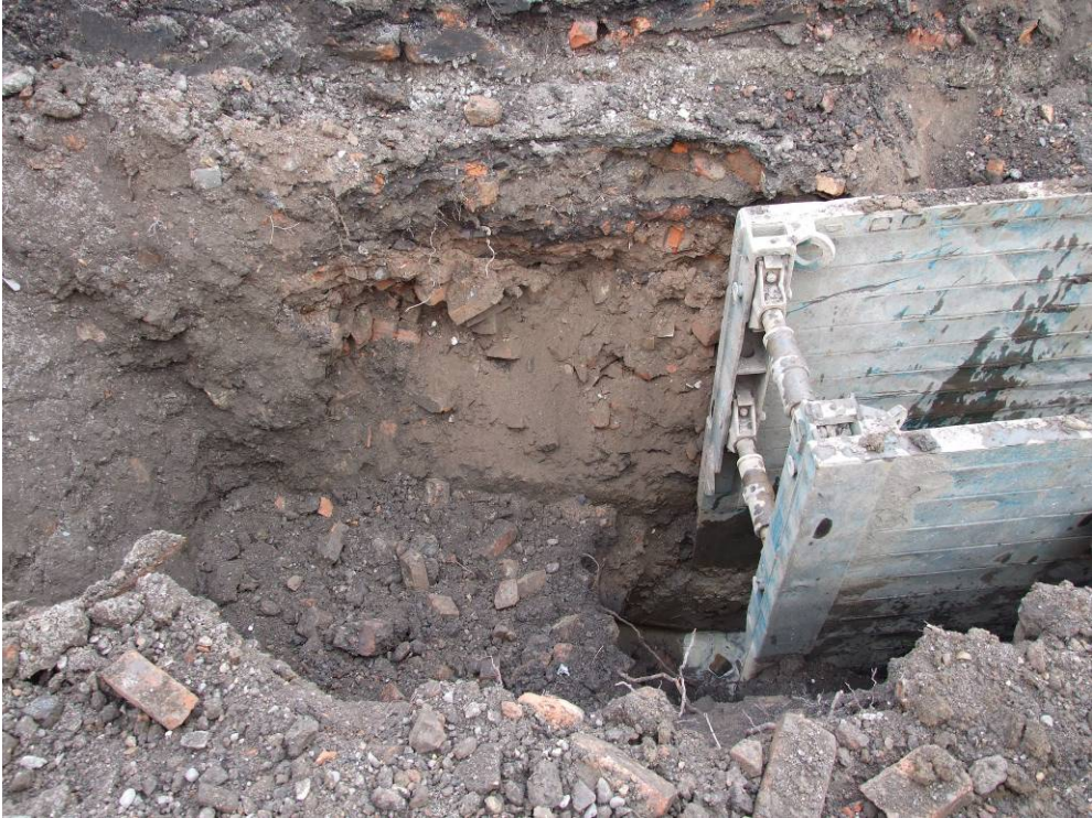
Plate 13: Made ground deposits within deep excavation
