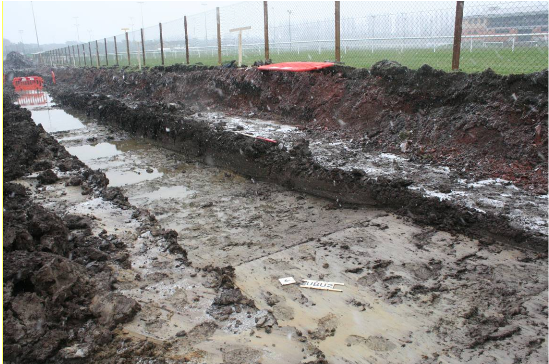
Plate 7: University Boulevard: East facing view of Environmental Trench 18.
