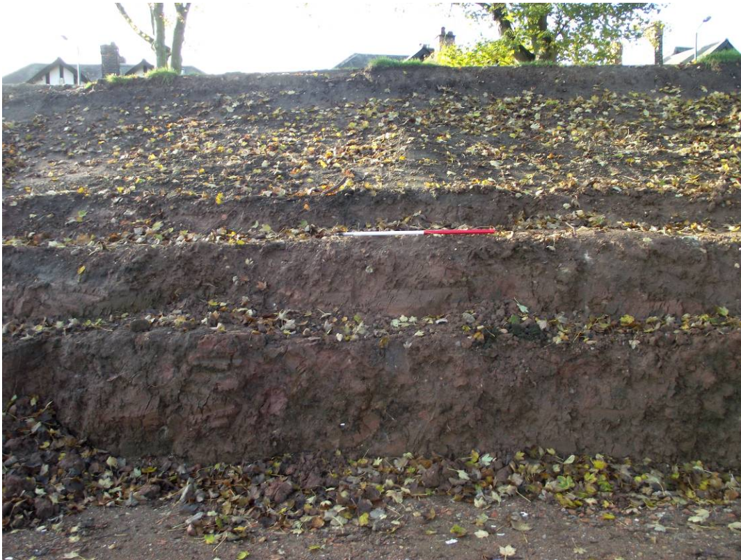
Plate 25: Section of disused Great Northern Railway embankment (WCA0001) and (WCA0002)
