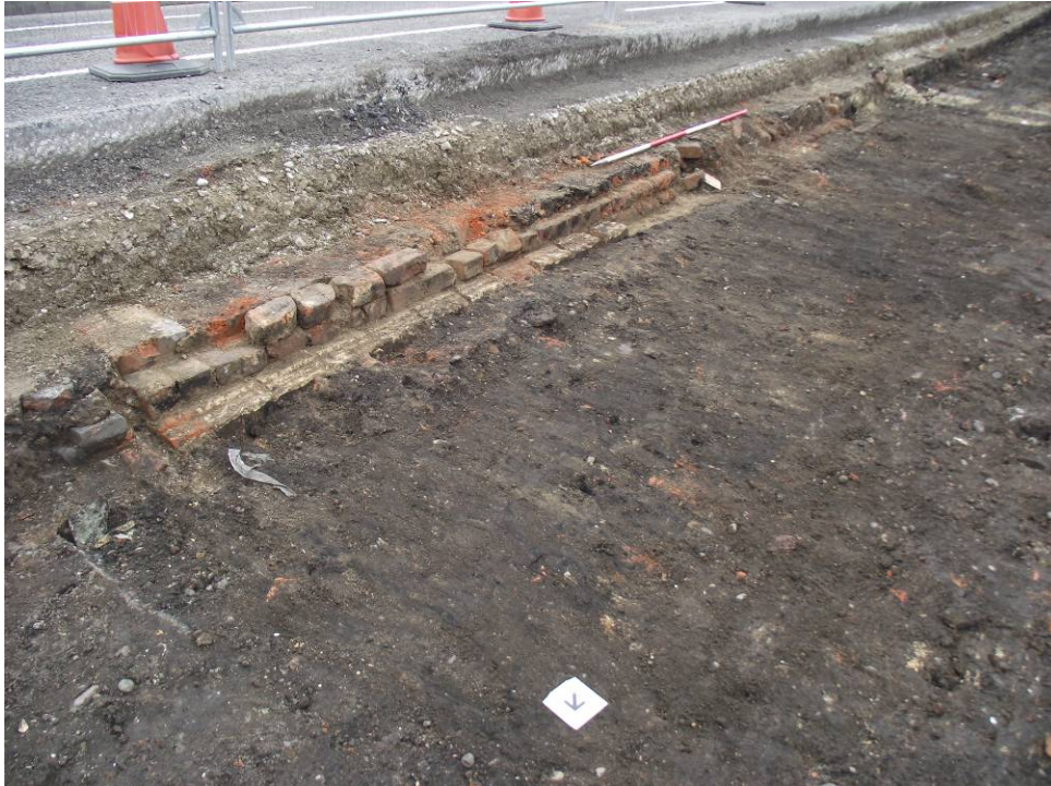
Plate 18: Meadows Way: Linear 19 th century wall (MWN0059). Possible industrial structure. Looking South.
