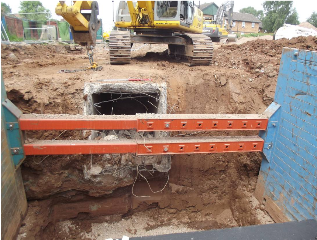
Plate1: Chilwell: Bisected Culvert (CED0008) near Greenwood Court.
