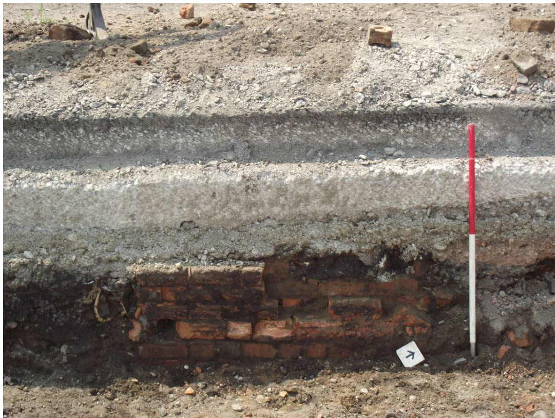
Plate 20: Meadows Way: Five courses of red brick, 19 th century wall (MWN0068) not visible in plan and ceramic drain (MWN0069). Looking Northwest.
