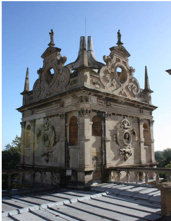
External view of the South-east corner tower
