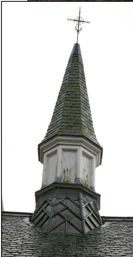
Plate 8: Detail of the octagonal flèche, viewed looking east.
