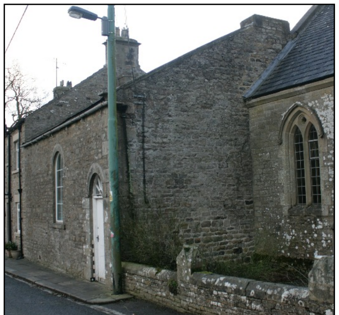
Plate 3: The possible former bellcote in the north gable wall of the Sunday School, viewed looking south-west.
