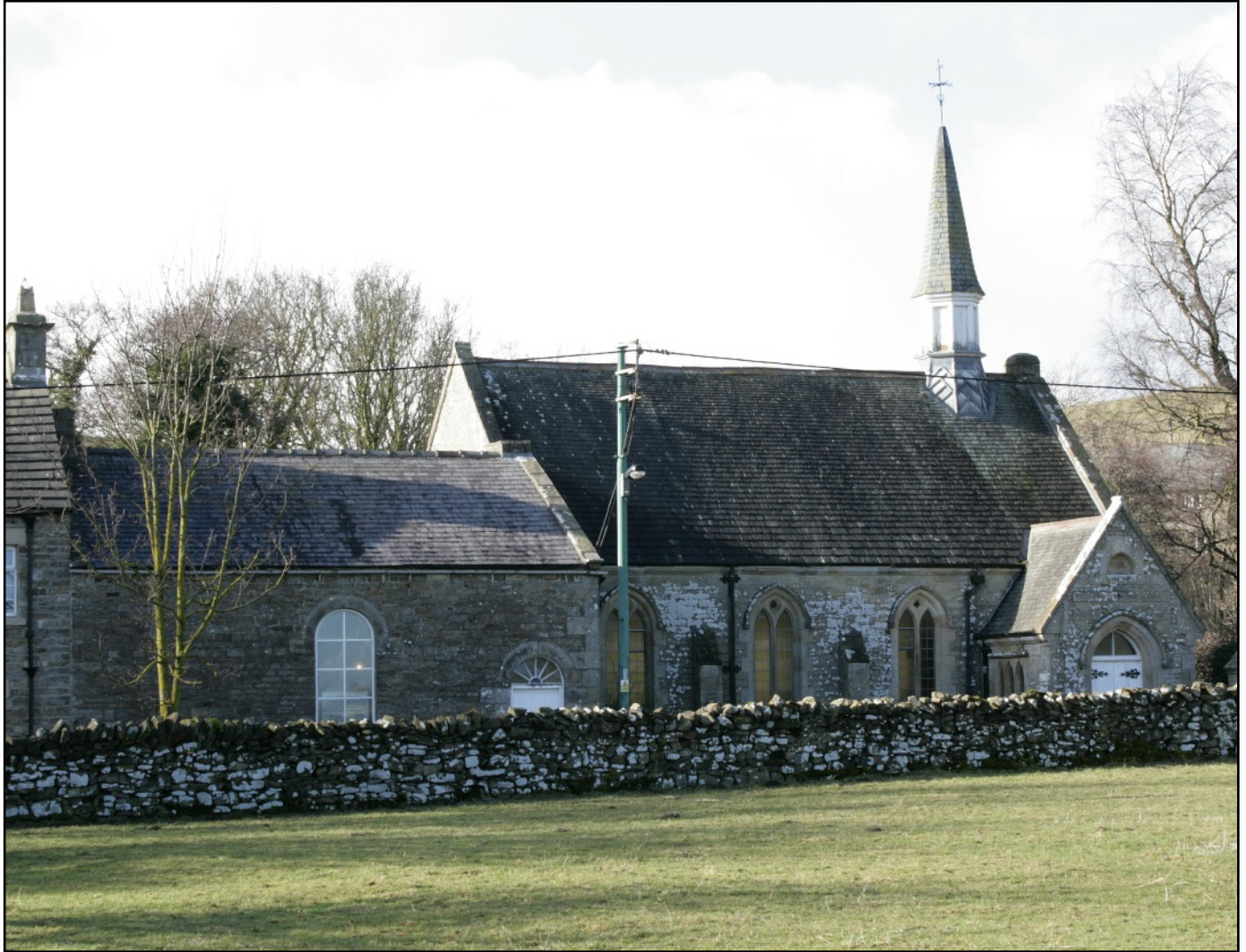
Plate 1: General view of the Wesleyan Methodist Church at Eastgate with the earlier phase of c. 1819 to the left and the later Gothic style Cuthbert Memorial Wesleyan Chapel of 1891 to the right. Viewed looking north-west.
