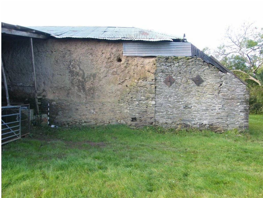
Plate 2: Northeast elevation of the threshing barn and shippon, viewed looking southwest
