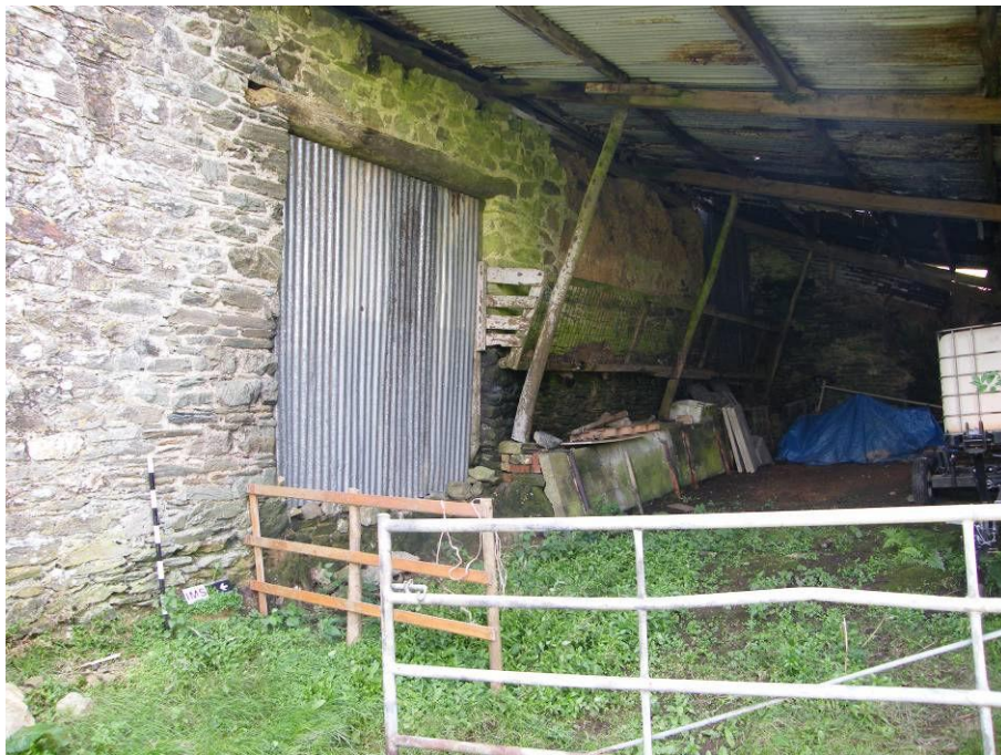
Plate 6: Cart door in the southwest elevation, viewed looking southeast
