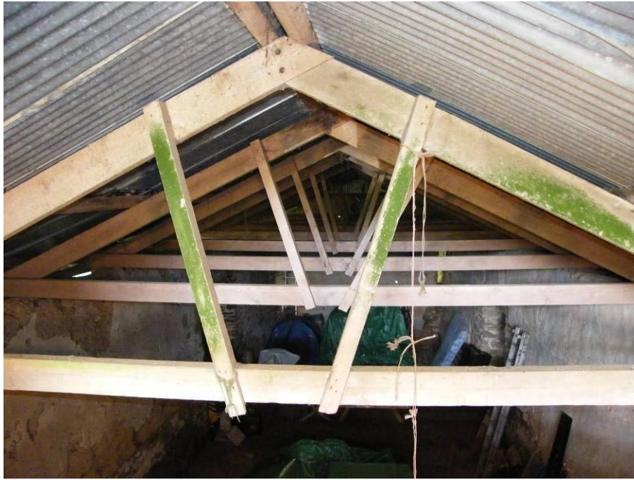
Plate 9: General view of the roof, viewed looking northwest
