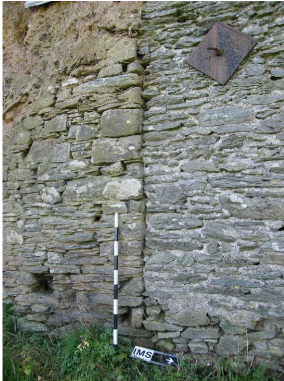
Plate 3: Building joint between the threshing barn and shippon on the northeast elevation, viewed looking southwest
