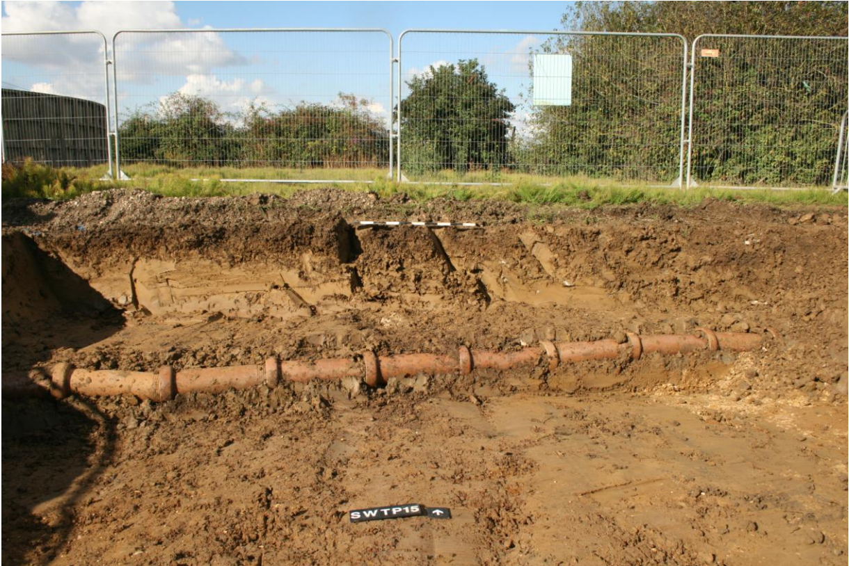
Plate 3: South facing section, looking north
