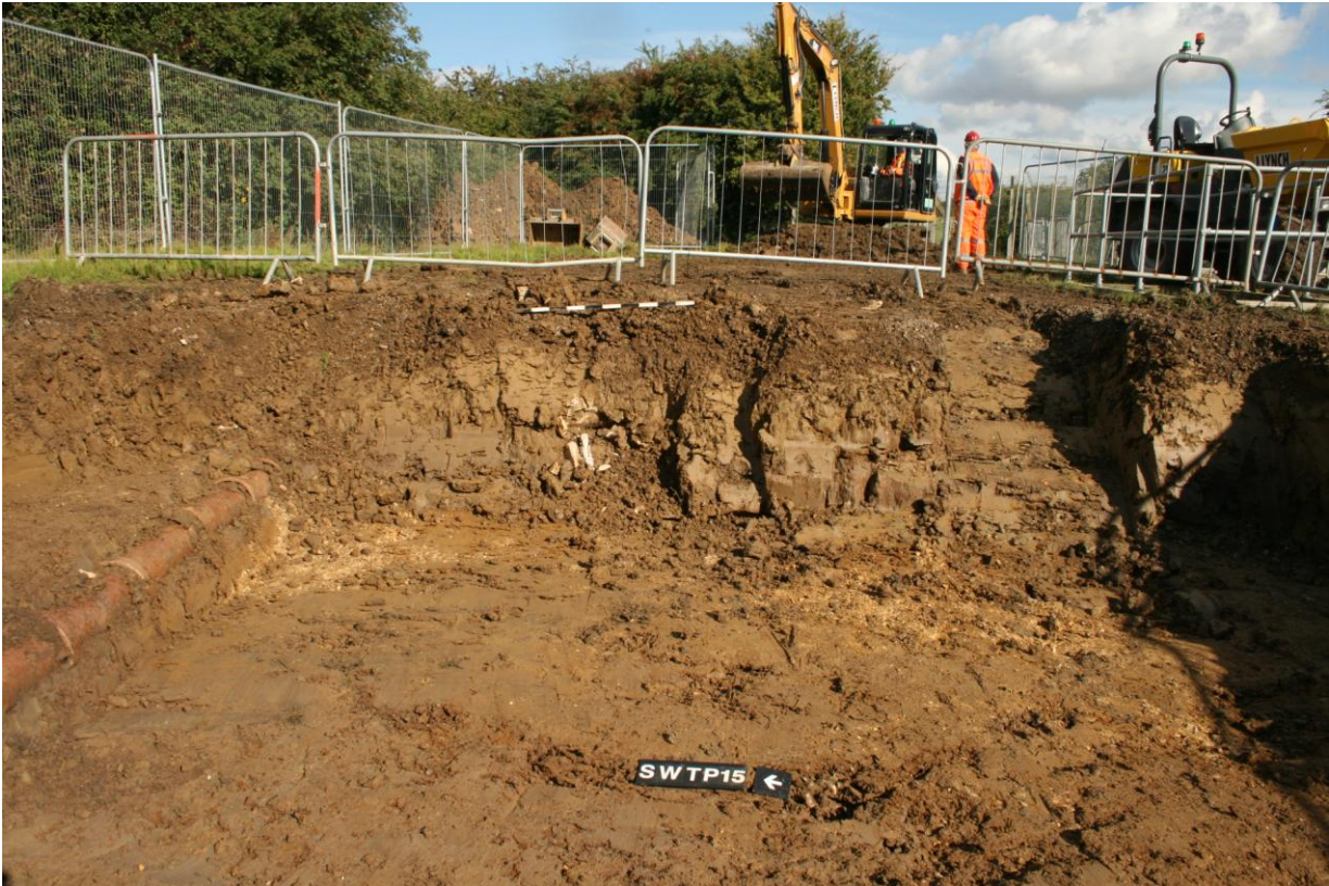
Plate 4: View of the east facing section with access ramp, looking west
