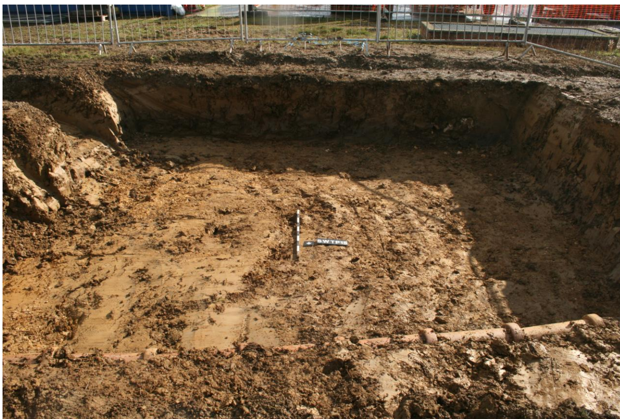
Plate 5: General view, looking south
