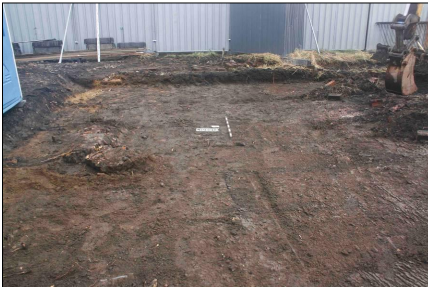
Plate 4: South End of Trench 1, after the removal of the 1912 footings
