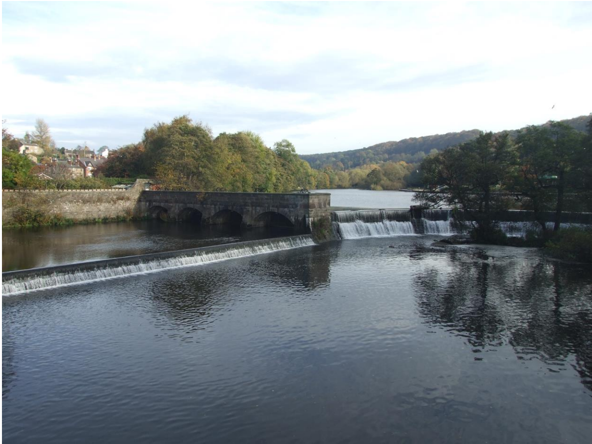
Figure 2: The Horseshoe Weir, built by Jedediah Strutt to power the West Mill at Belper. Construction commenced in the last decade of the 18 th century. The weir was heightened and modified in 1819 and 1843 but remains substantially unaltered. Photograph: D. Knight
