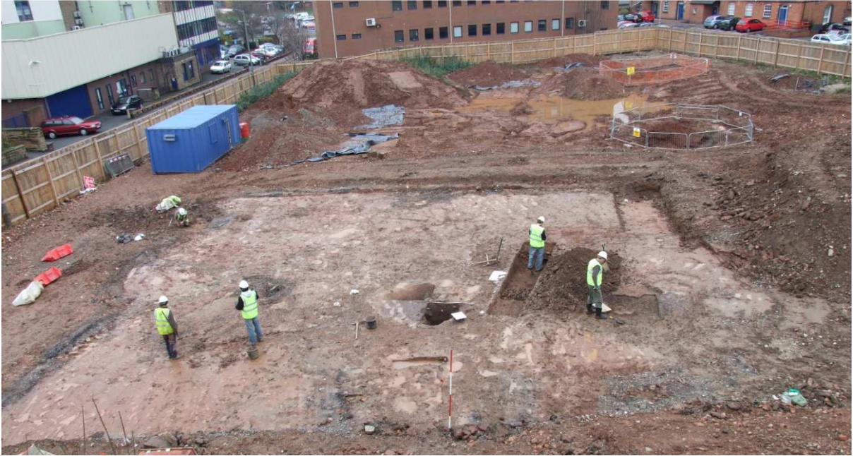
Plate 1: General view, excavation in progress Area 25
