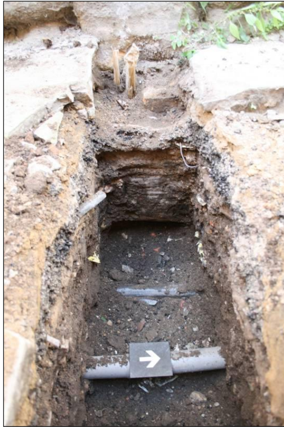
Plate 5: Foundations for chapel
