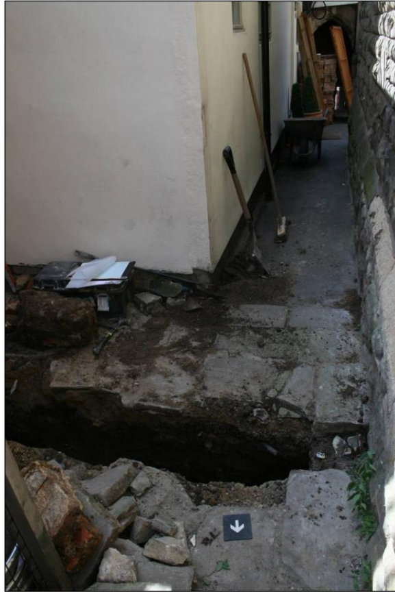
Plate 3: Post excavation, general shot
