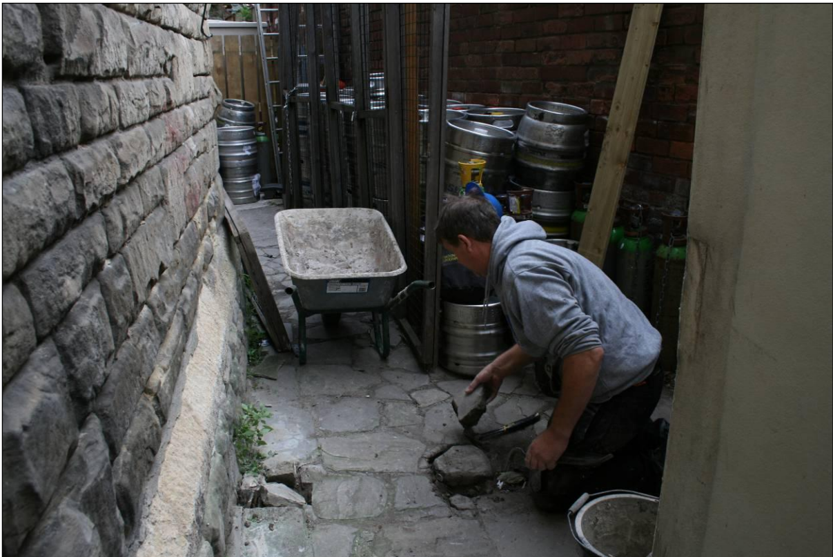
Plate 1: Site prior to excavation, looking north
