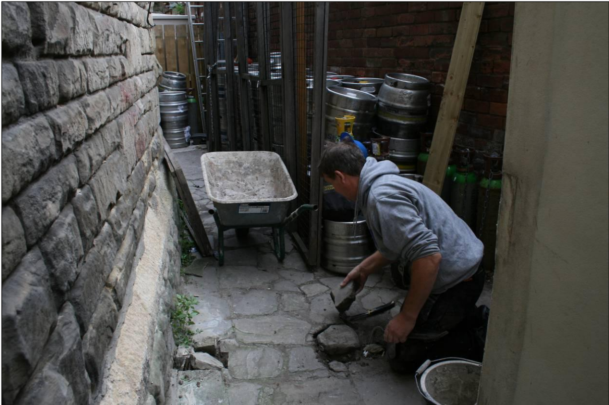
Site prior to excavation, looking north
