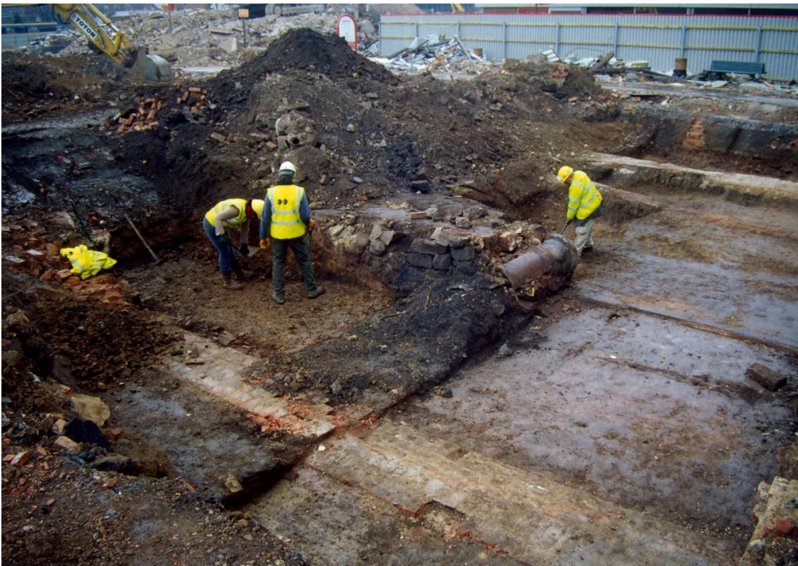
Plate 6 Cleaning in progress on the jetty structure in Area 09. Note the walls of the later works that had cut through the filled in tank/pool. Also, in the middle right is the thick clay lining of the tank/pool.
