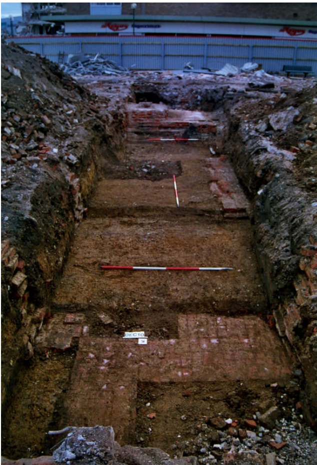
Plate 2 Area 10 evaluation trench showing brick floors in trench and walls in section.
