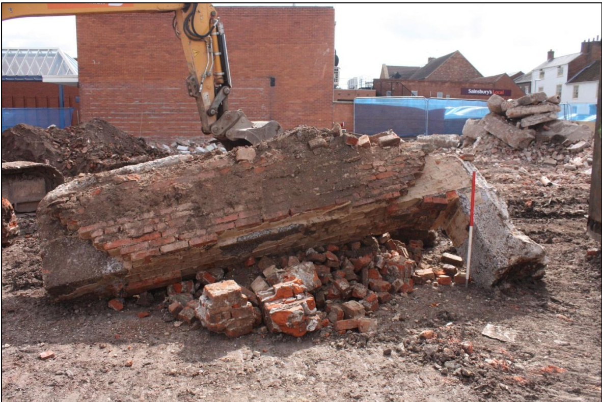
Plate 14. Concrete filled, brick lined corridor that once adjoined the cellar.
