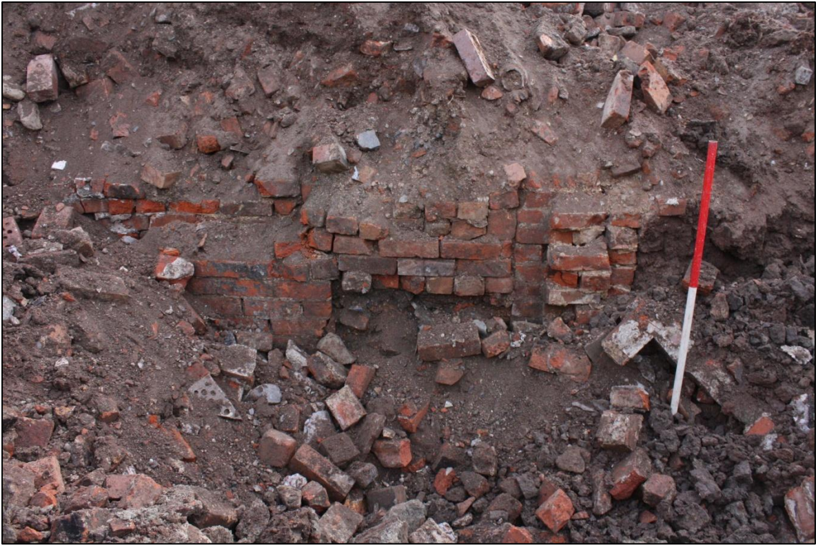
Plate 15. Close-up detail of bricked-up entrance within eastern wall of coal cellar viewed looking east.
