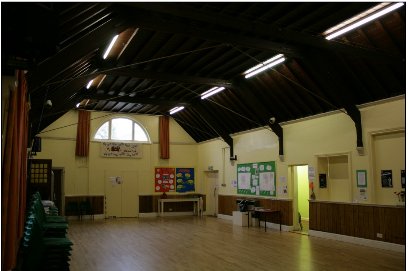
Plate 12. The interior of the earliest phase of the Sunday School viewed looking north east.
