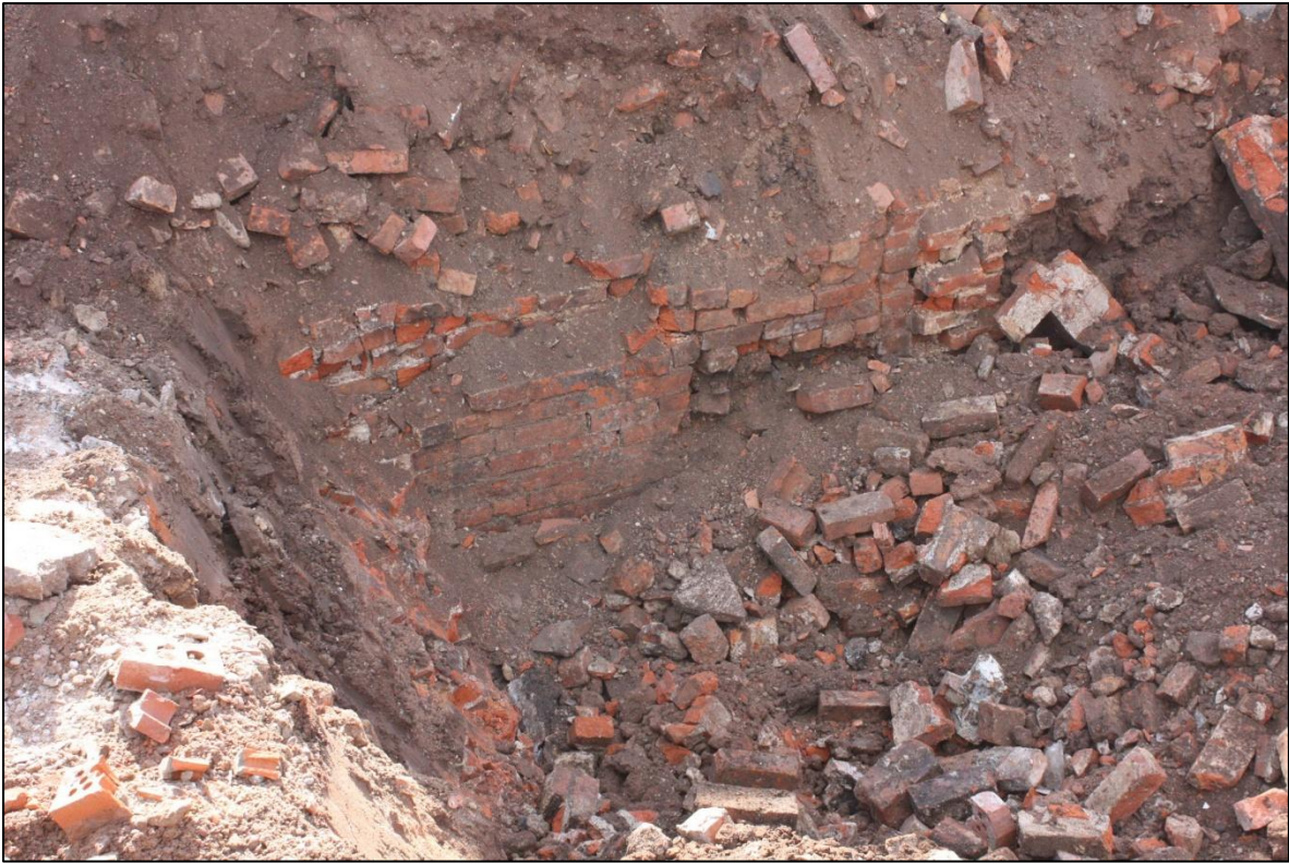
Plate 13. Eastern wall of coal cellar, with bricked-up entrance, viewed looking south east.
