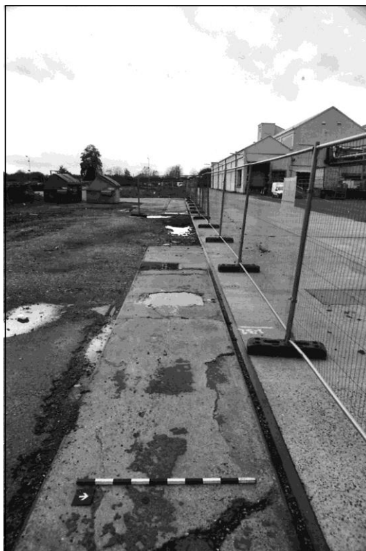
The rail sidings of Sixth Avenue extending towards D1
