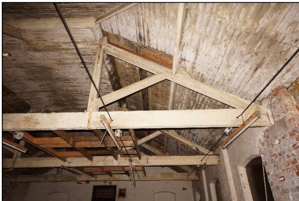
Plate 11: The roof over Phase D viewed looking south-west.
