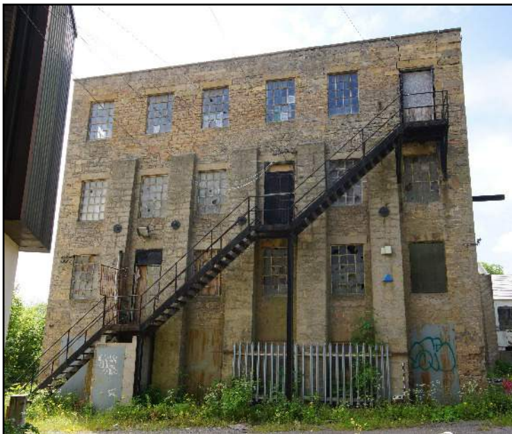
Plate 15: The north elevation of Phase G, viewed looking south.
