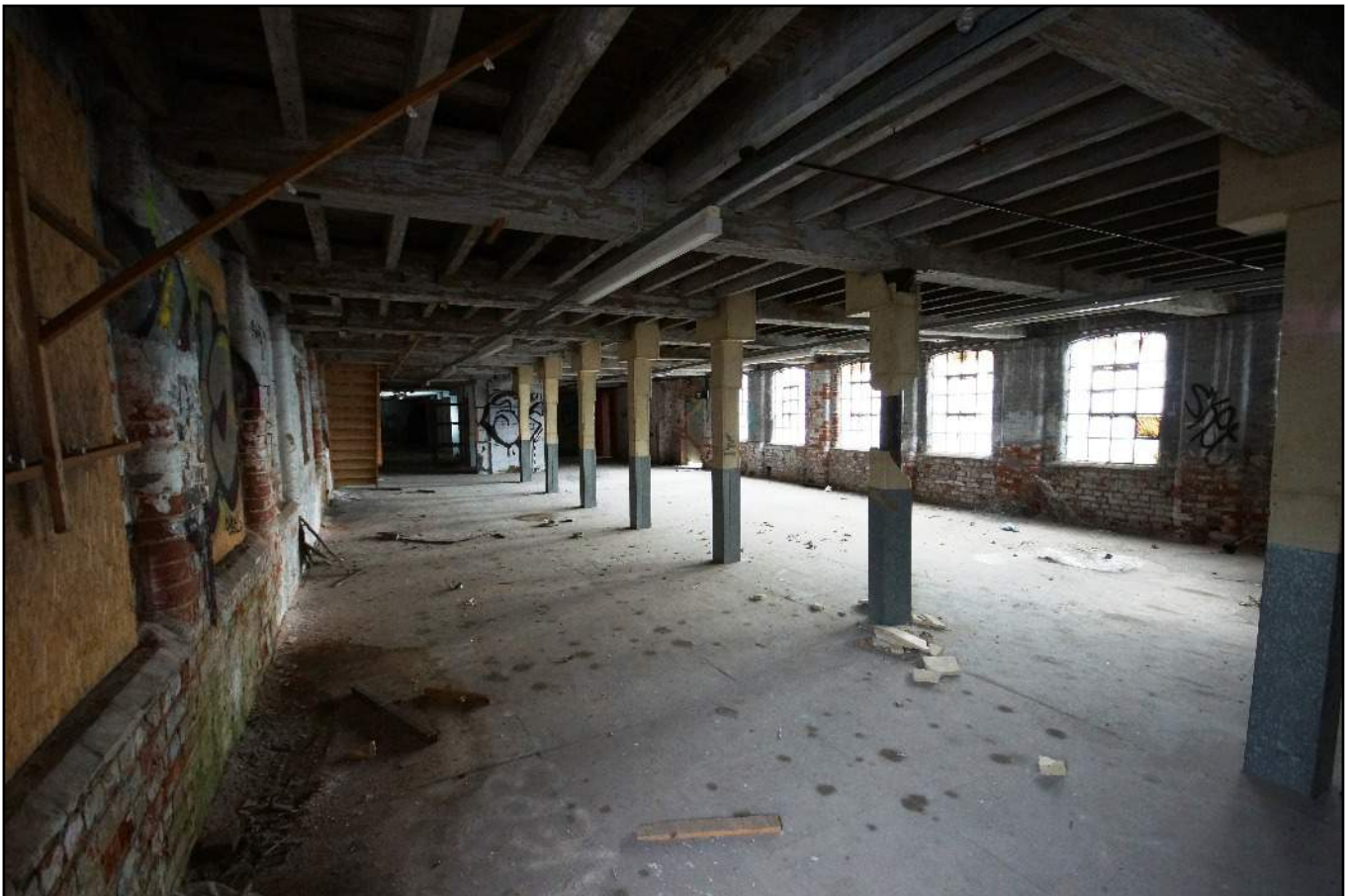
Plate 13: The upper ground floor of Phase E, viewed looking north-east.
