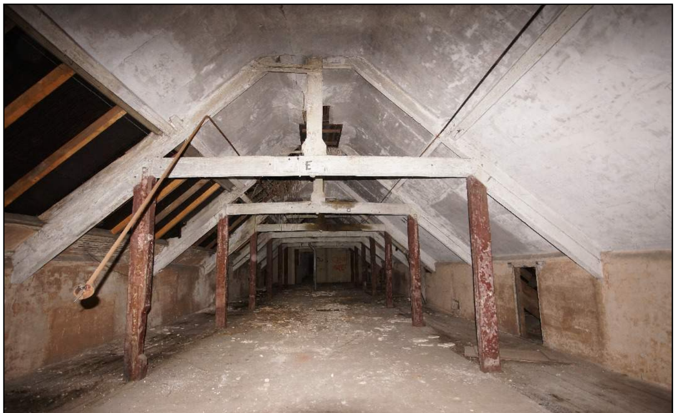
Plate 4: General view of the roof of Phase A, viewed looking south.
