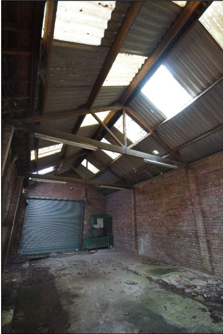
Plate 17: The interior of the Phase I, viewed looking south-west.
