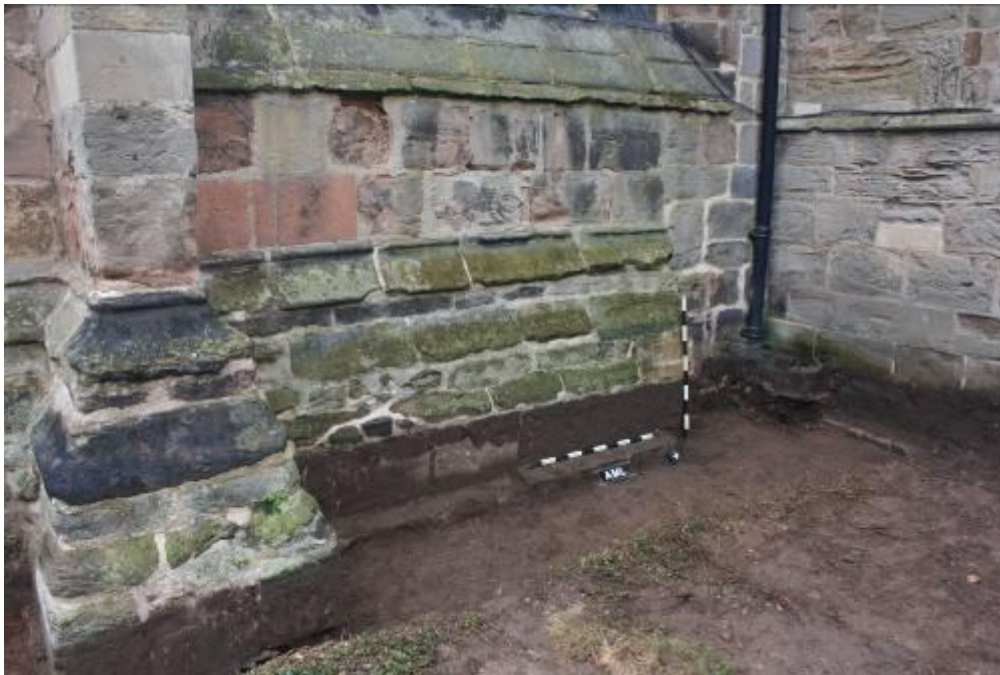
Plate 9. Area 02 showing exposed foundations. Looking north west.
