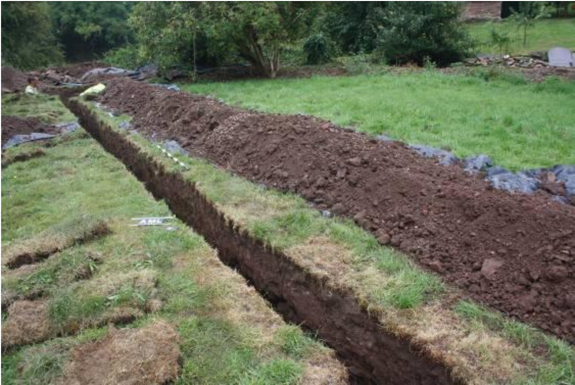
Plate 21. Area 08. Drainage trench overall view. Looking east.
