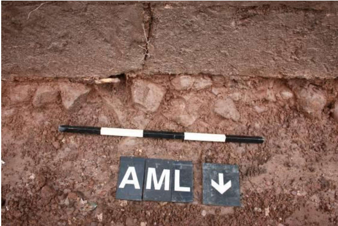
Plate 17. Area 05. Detail of pebble foundation of north facing wall of Appleby Chapel. Looking south.
