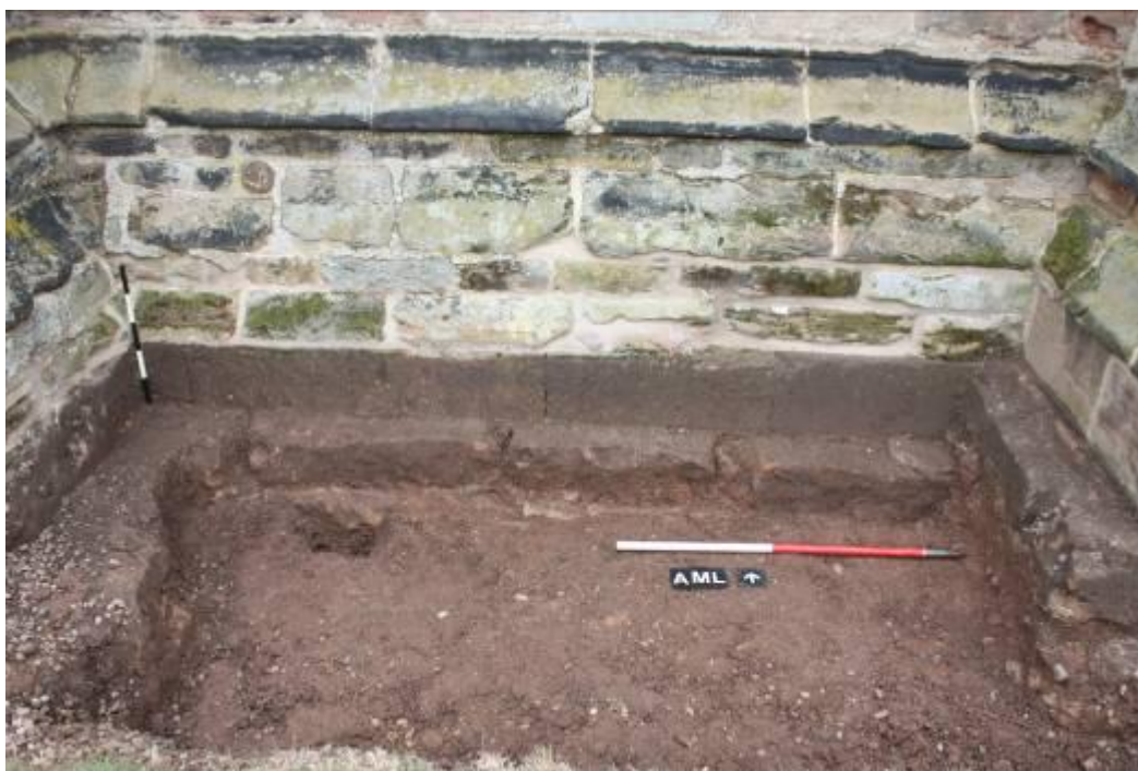
Plate 5. Area 01. Detail of excavation along the south of the church showing exposed foundations. Looking north.
