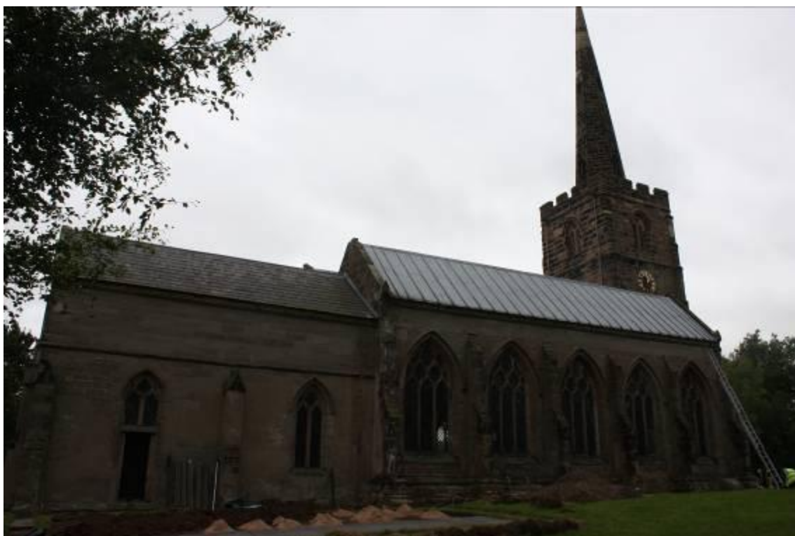
Plate 3. North facing wall of the Appleby Chapel and north aisle. Looking south west.
