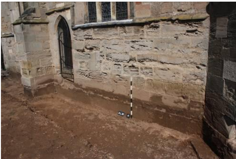
Plate 10. Area 03 showing top of foundation. Looking north west.
