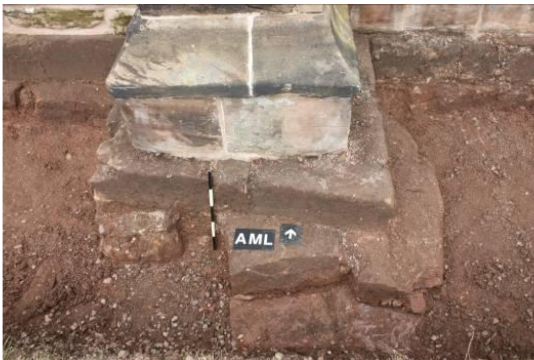
Plate 6. Area 01. Two slabs protruding from beneath the foundation of the buttress. The south porch is believed to have been situated in the bay to the left of the buttress. Looking north.
