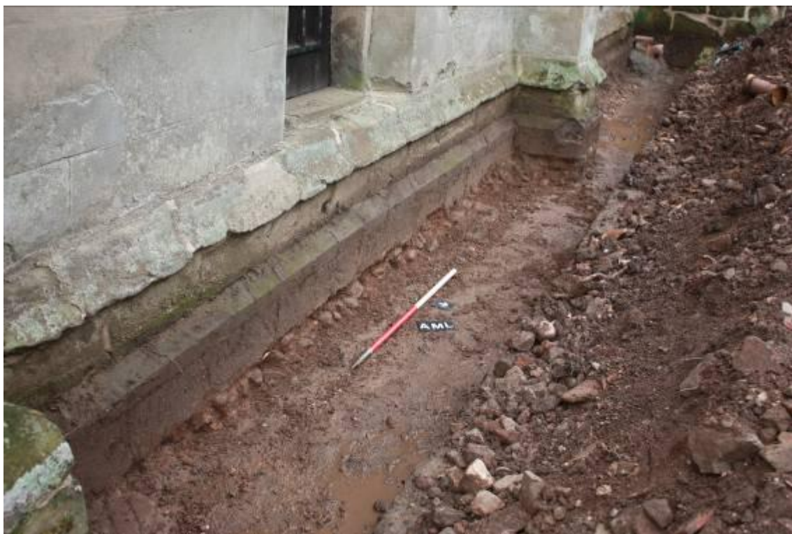
Plate 16. Area 05. Oblique view of north facing wall of Appleby Chapel showing pebble foundation. Looking south west.
