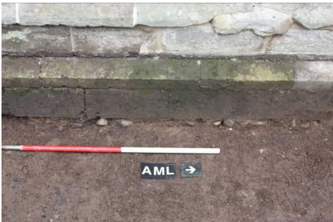
Plate 14. Area 04. Detail of pebble foundation of east facing wall of the Appleby Chapel. Looking west.
