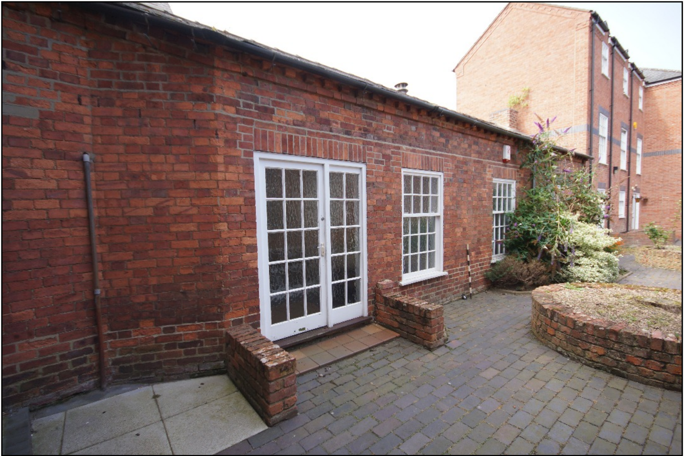
Plate 21: The east elevation of the West Range, viewed looking north-west.
