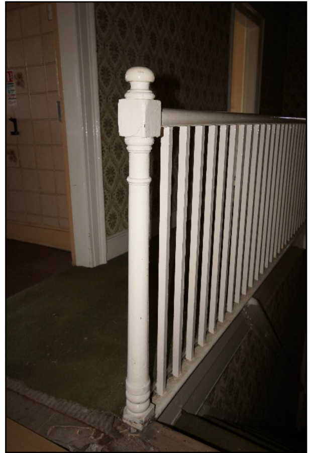
Plate 18: The bannister in Hallway 39, viewed looking south-west.
