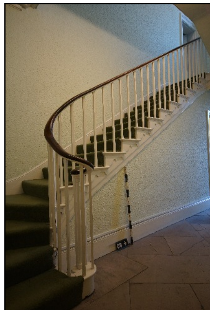
Plate 14: The staircase in Hallway 08, viewed looking north-west.
