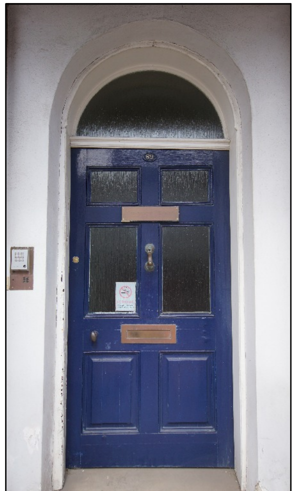
Plate 3: The door in the south frontage, viewed looking north.
