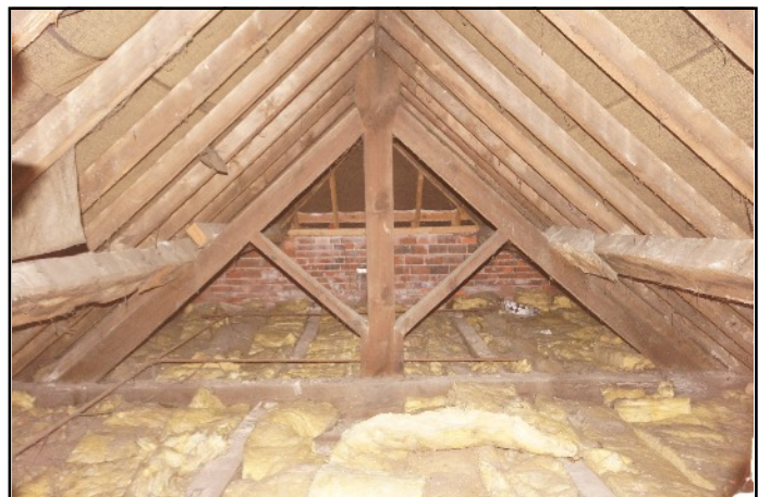
Plate 20: The king post roof over Room 26, viewed looking north.
