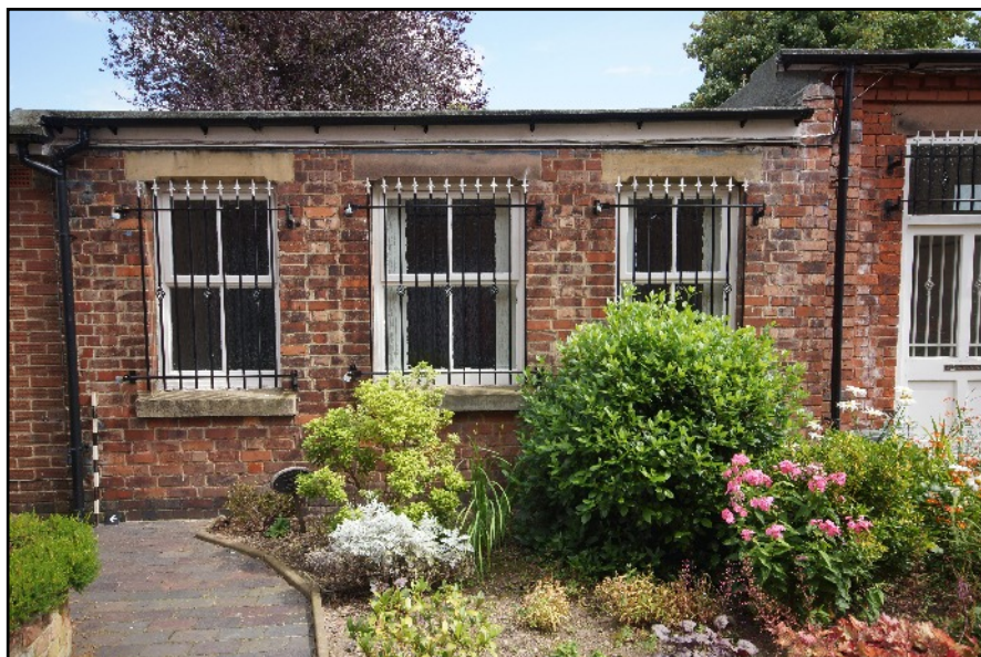
Plate 26: The west elevation of the East Range Phase III, viewed looking east.
