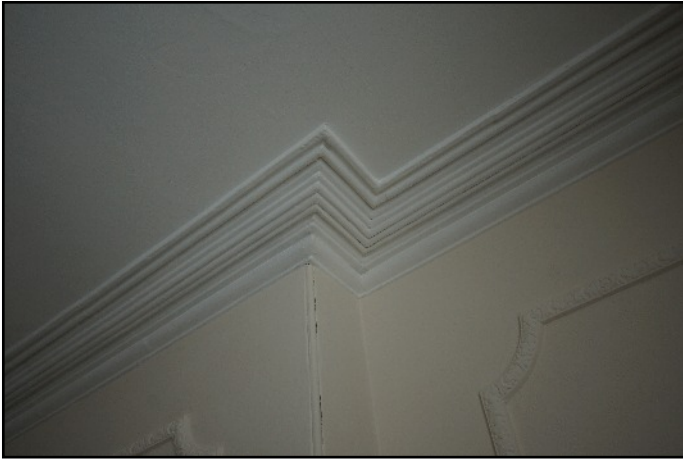
Plate 15: The plaster cornice in Room 25.
