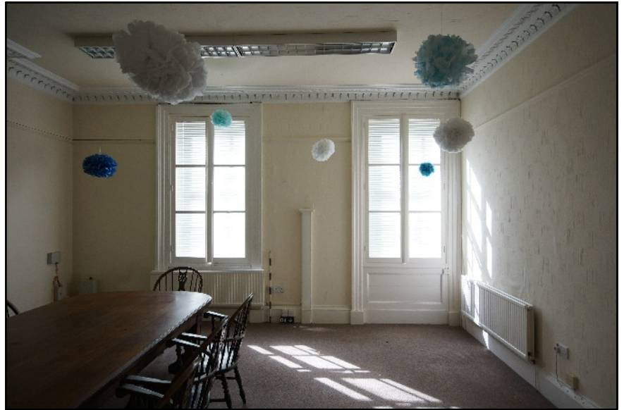
Plate 10: General view of Room 04, viewed looking south. Note the surviving boxes for the shutters beneath the windows.
