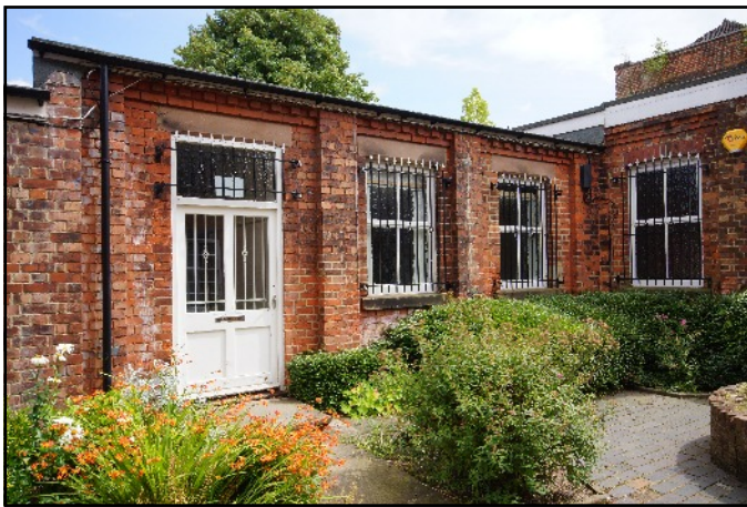
Plate 24: The west elevation of the East Range Phase II, viewed looking south-east.
