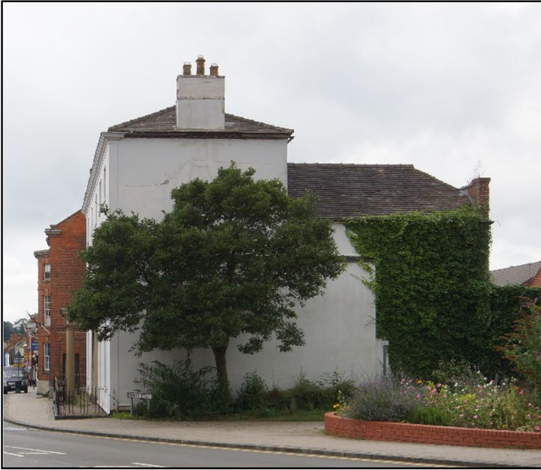
Plate 4: The east gable and elevation of the north element of St. Helen's House, viewed looking west.
