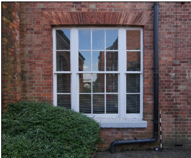
Plate 8: The ground floor window in the north elevation, viewed looking south.
