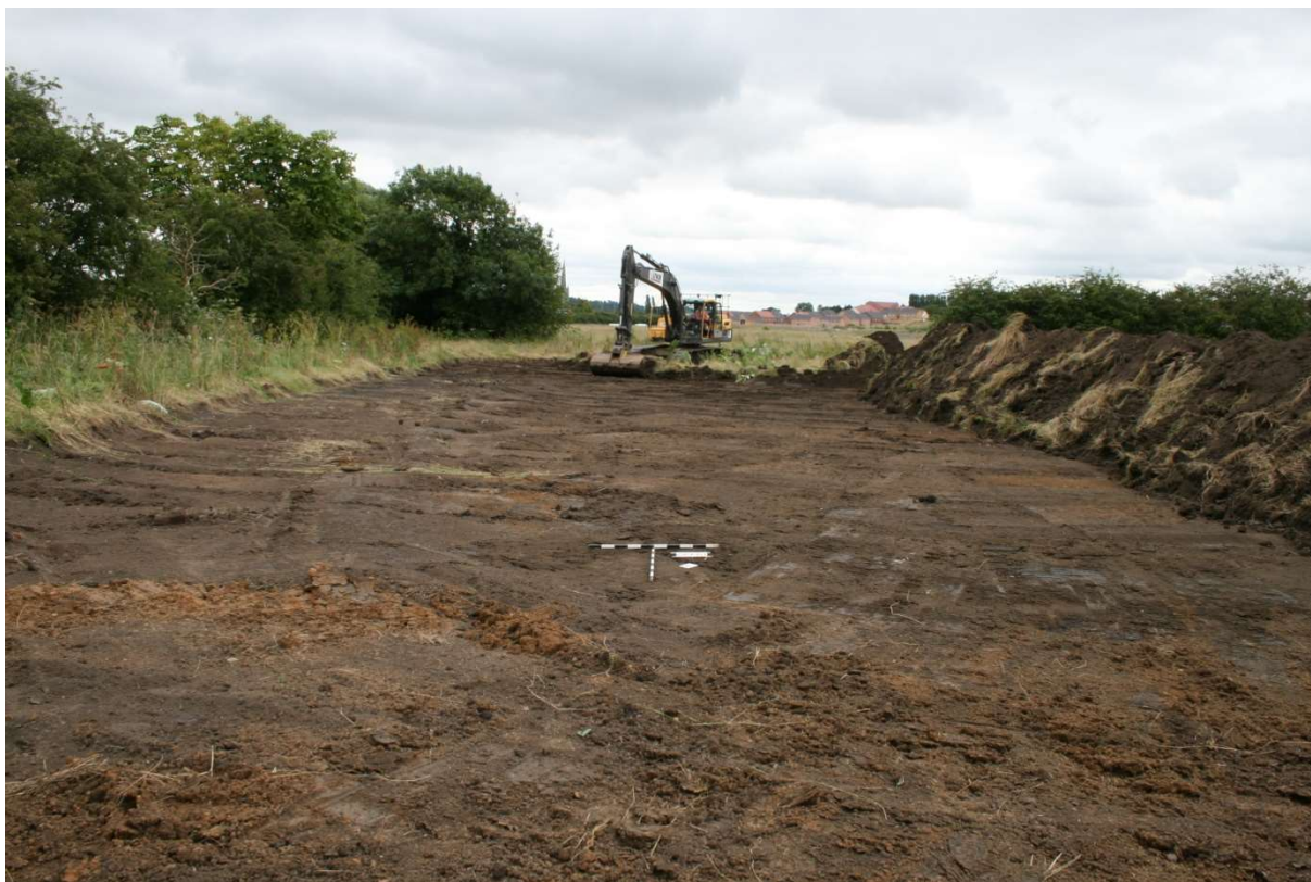
Plate 1: The site strip underway, looking south-east
