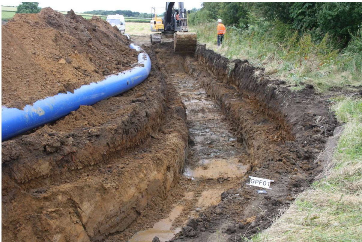
Plate 3: The north-eastern portion of the trench during excavation, looking north-west.
