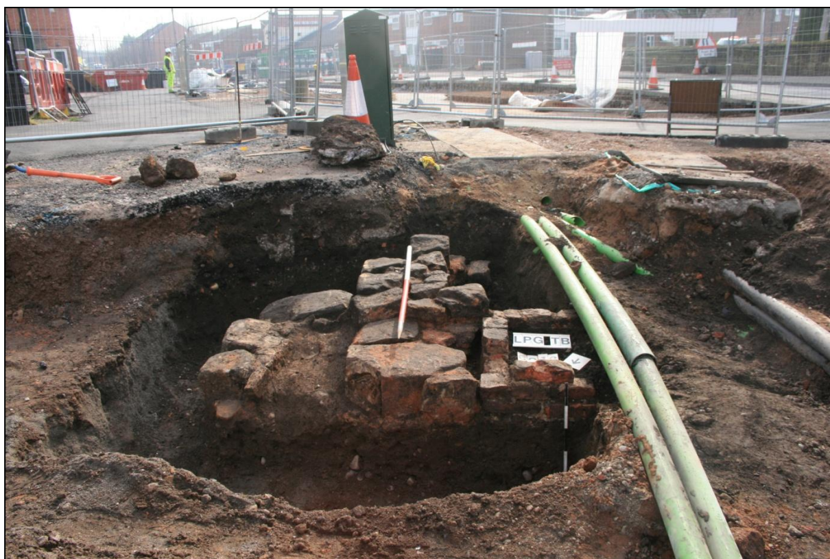
Plate 23: Stonework found near to the site during NET2 works Looking southeast. (TPA 2012)
