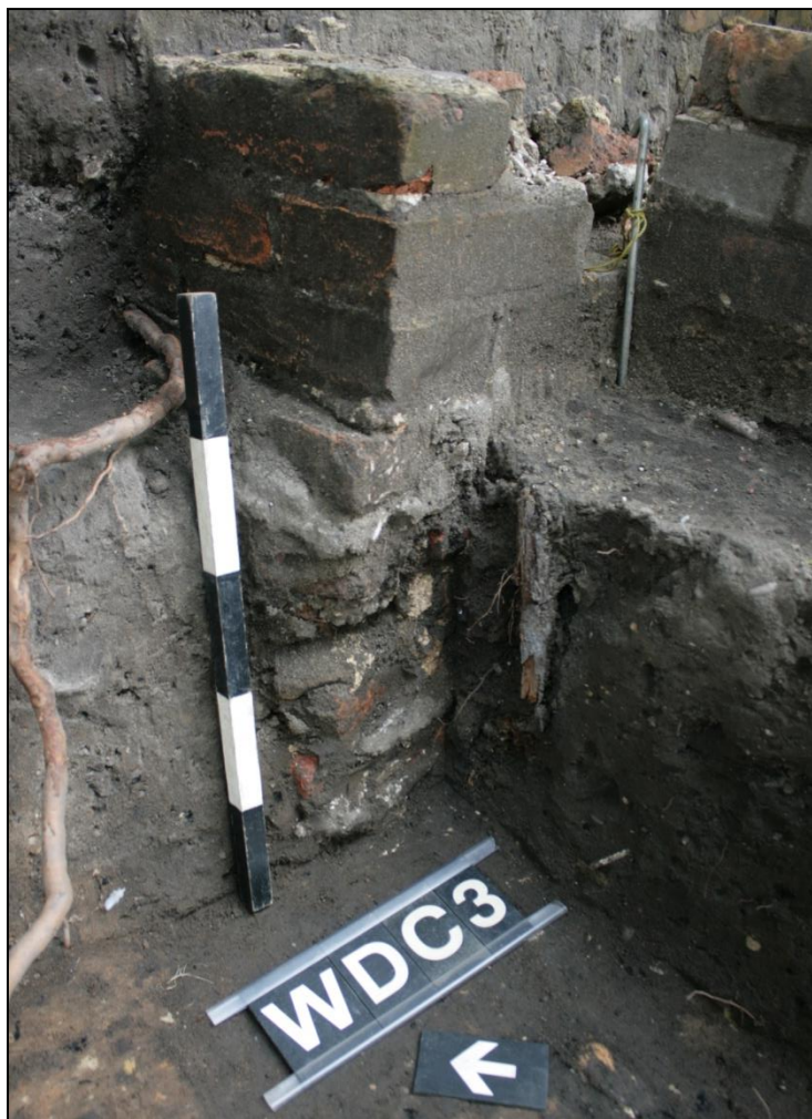
Plate 58 (Left): Wall [0222] protruding beyond structure [0126]. Looking east (Trainees 2017)
