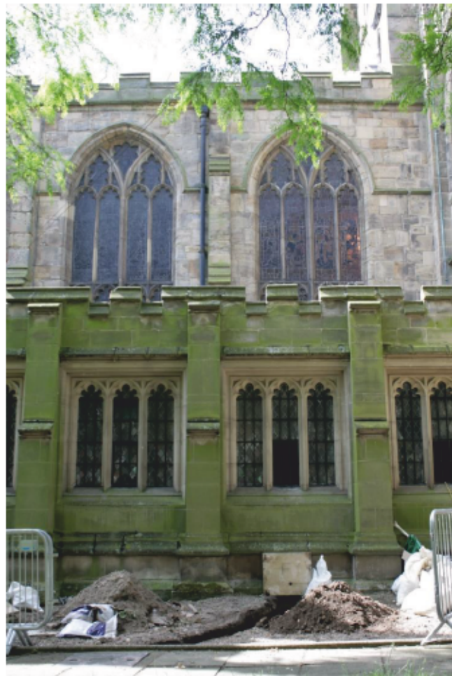
Plate 2: General view of the trench and Chapter House, viewed looking south.
