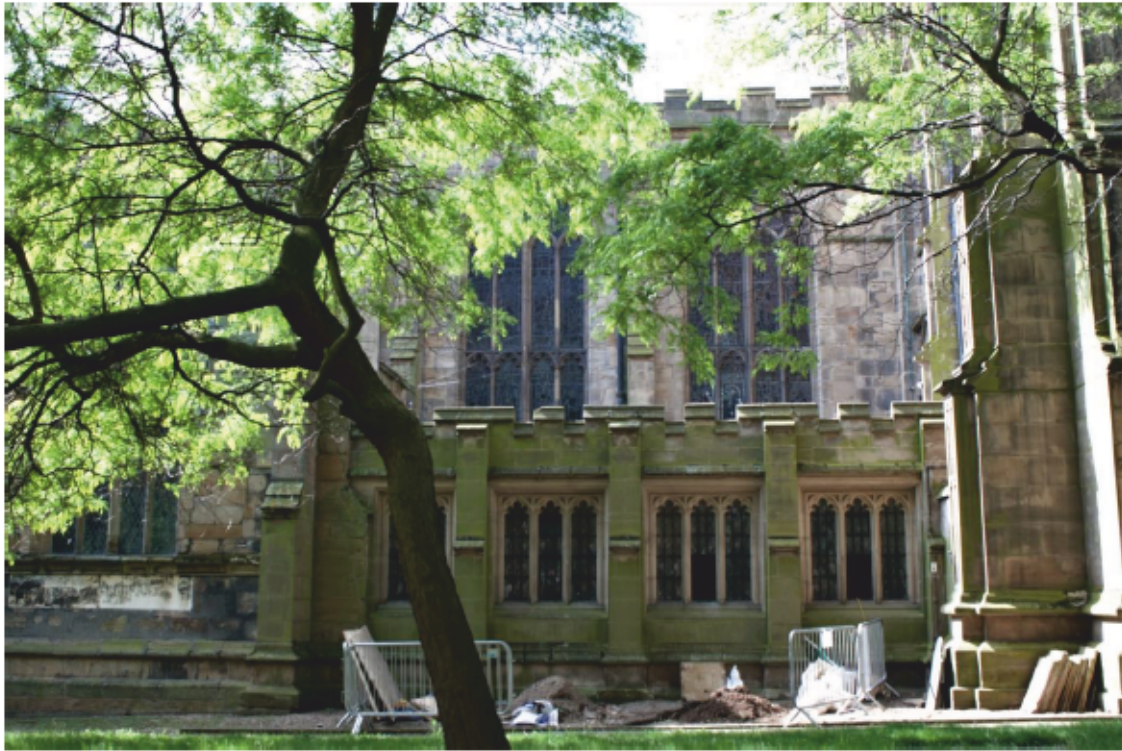
Plate 1: General view of site showing the trench and Chapter House, viewed looking south.
