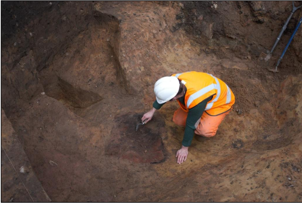
Plate 5: Working shot, looking northeast, of area over burnt area [0236] and posthole [0243] being excavated. Ditch [0108], which can be seen running from the top left the image towards the middle of the bottom edge, partly truncates [0104].
