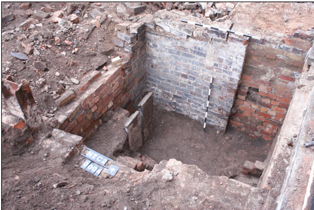
Plate 38: View of walls [0007] and [0008] in 'cellar' [0004], looking northwest, showing blue and red-bricks representing more than one structure. Fill partly excavated.
