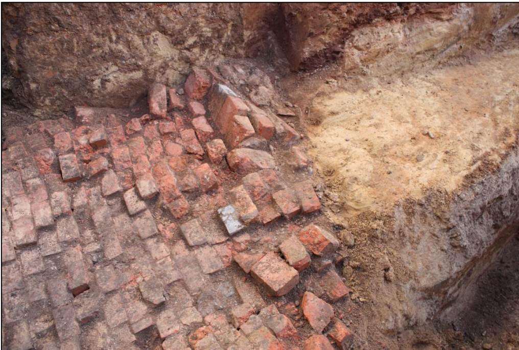
Plate 32: Detail of base of brick vault [0312], where it adjoins the bedrock on the southern side of the structure, showing the angled bricks in situ, with the rest of the vault having collapsed.
