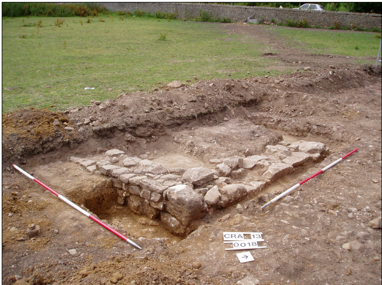
Plate 4 Area 13 showing post-medieval (c.17th century) structure interpreted as an outbuilding belonging to Bank House Farm. This was demolished in the 19th century
