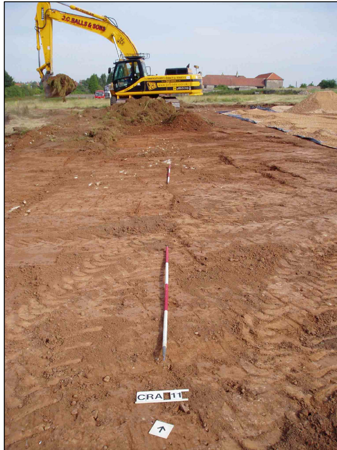
Plate 3 Area 11 stripping for compound works
