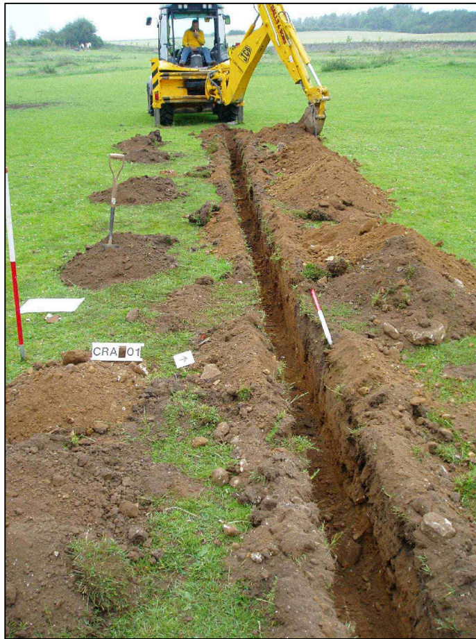
Plate 1 Area 01 enabling works. Water pipe trenching
